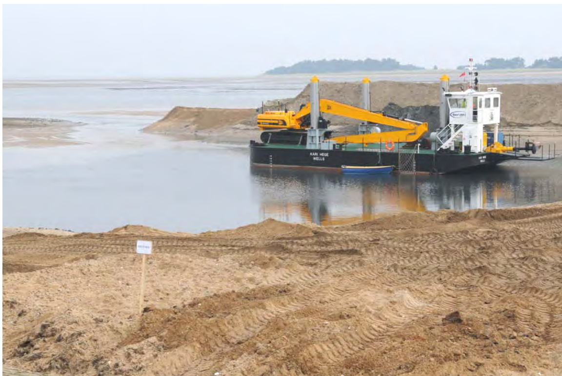
Figure IV.6 Dredging activities in Wells Harbour channel. Photo courtesy Claire Kinsley (North Norfolk District Council).
