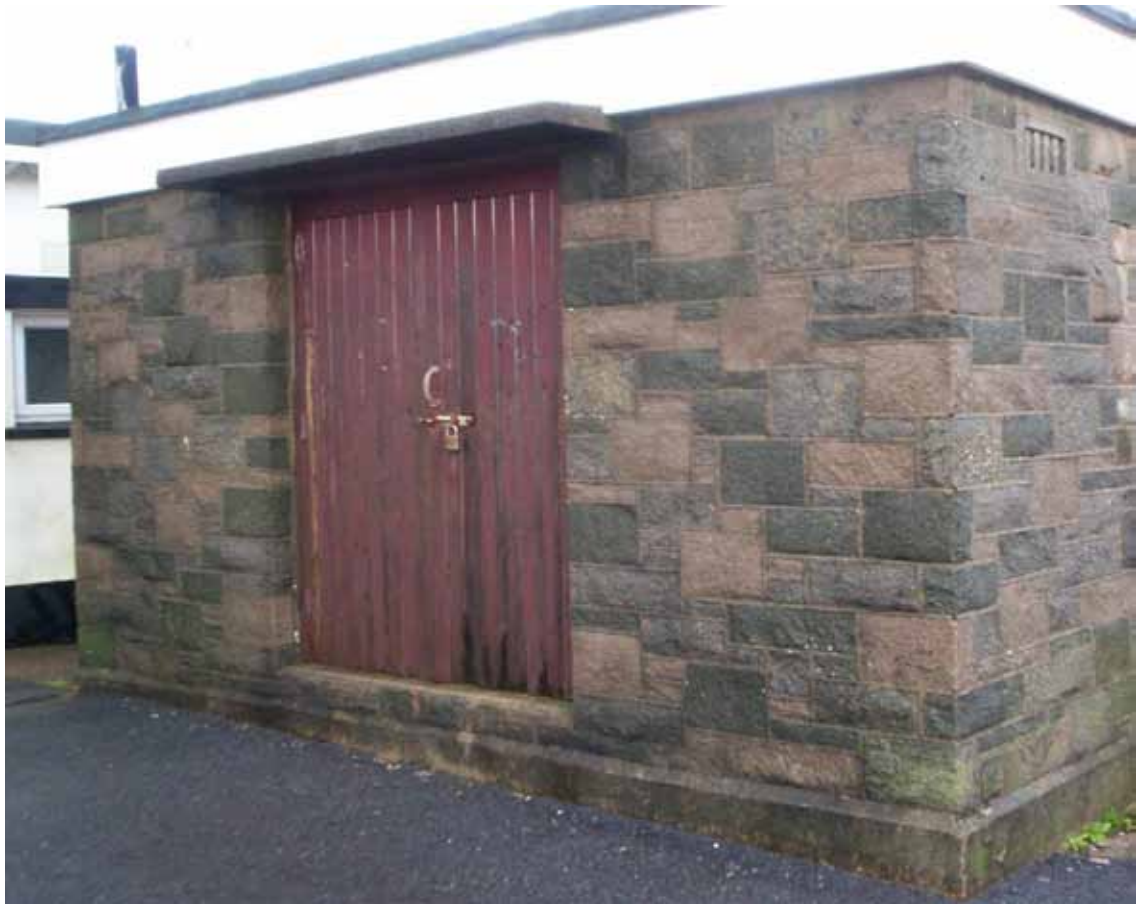
Figure XII.9 Stoke Gabriel Pumping Station.
