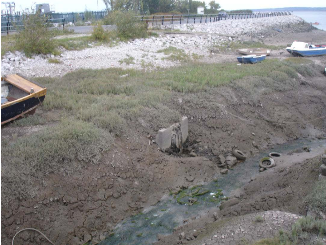
Figure XII.11 - Intermittent outfall to watercourse by Greenfield STW
