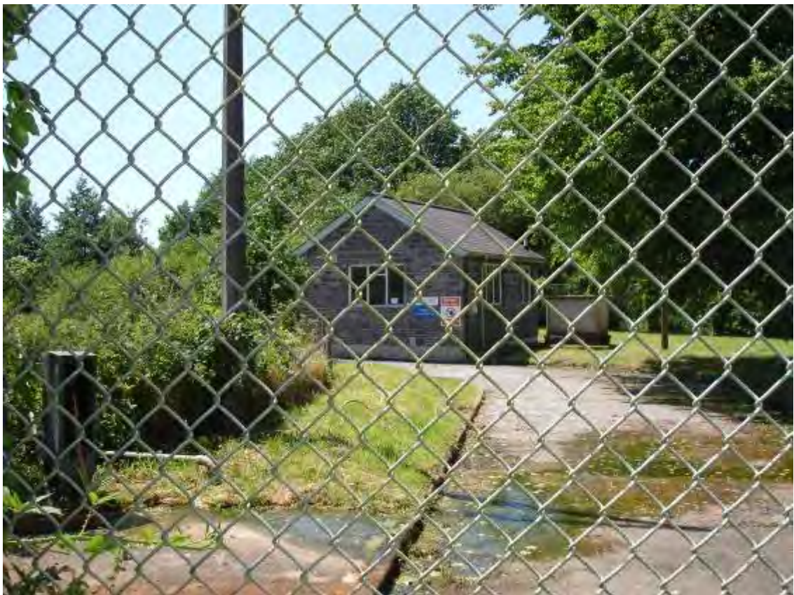
Figure XIII.6 Pennal sewage treatment works.
