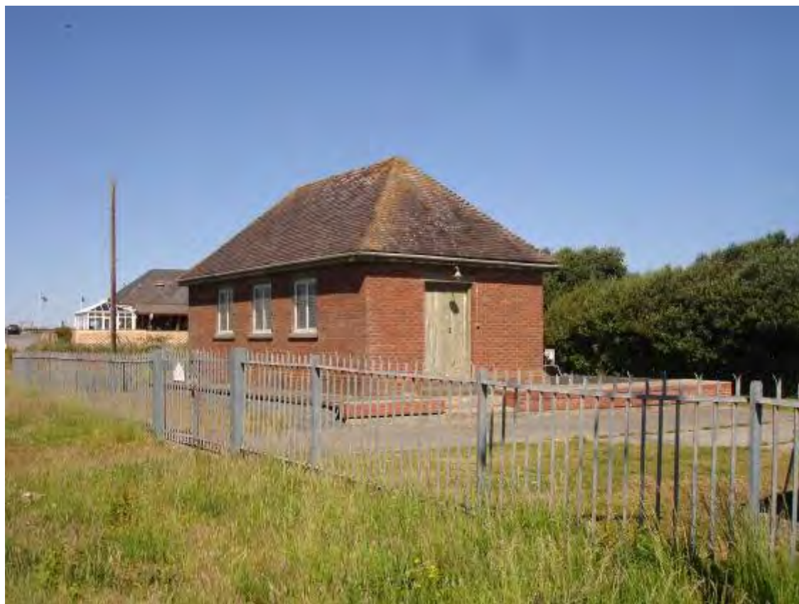
Figure XIII.4 Borth sewage treatment works.
