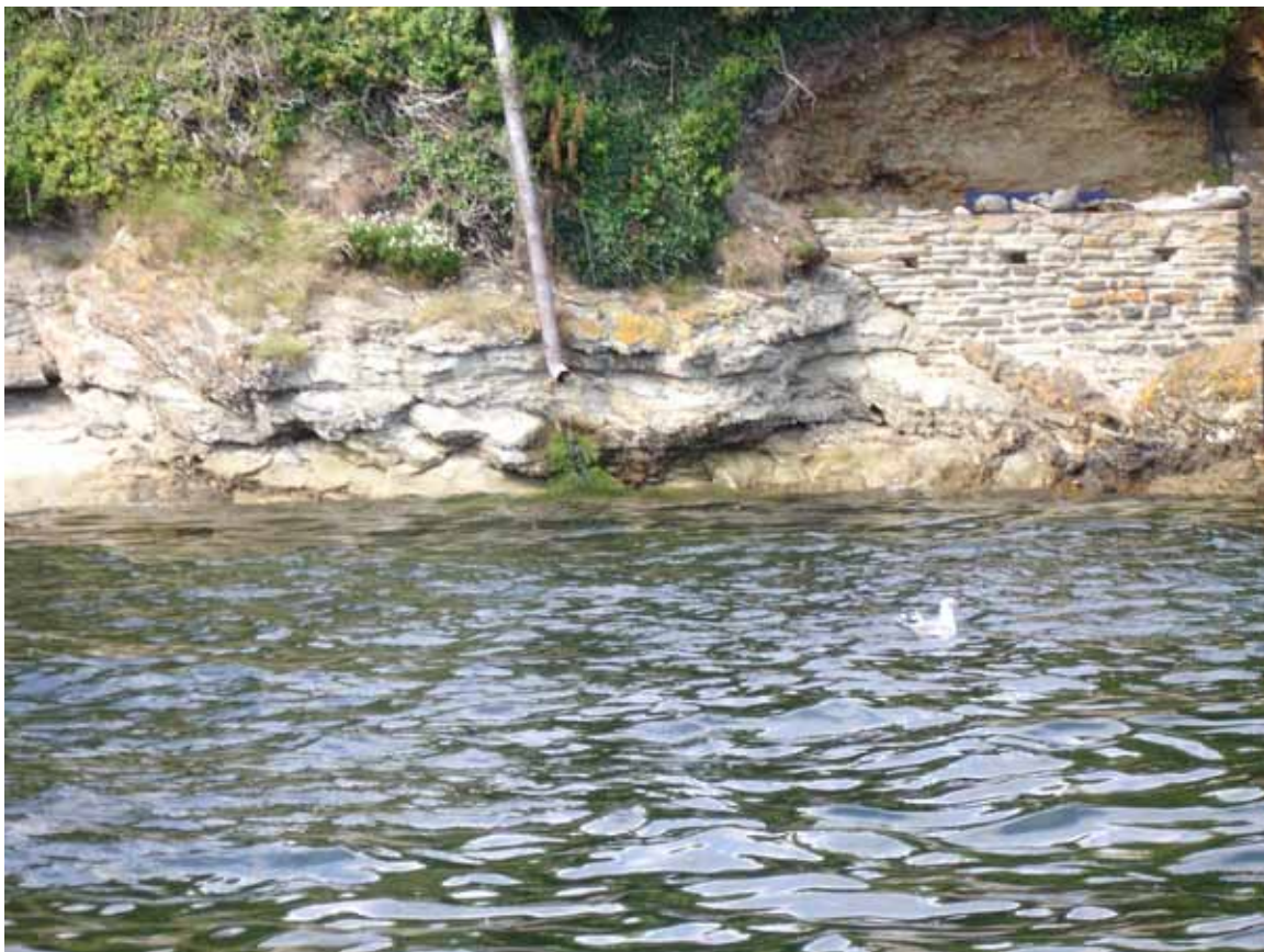
Figure XIII.12 Piped discharge at St. Just.
