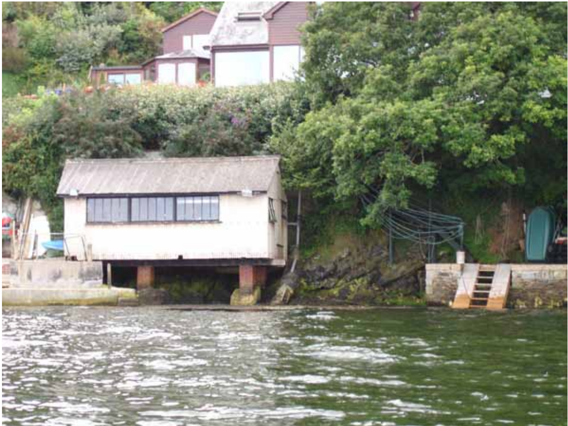
Figure XIII.11 Piped discharge at Weir Point.
