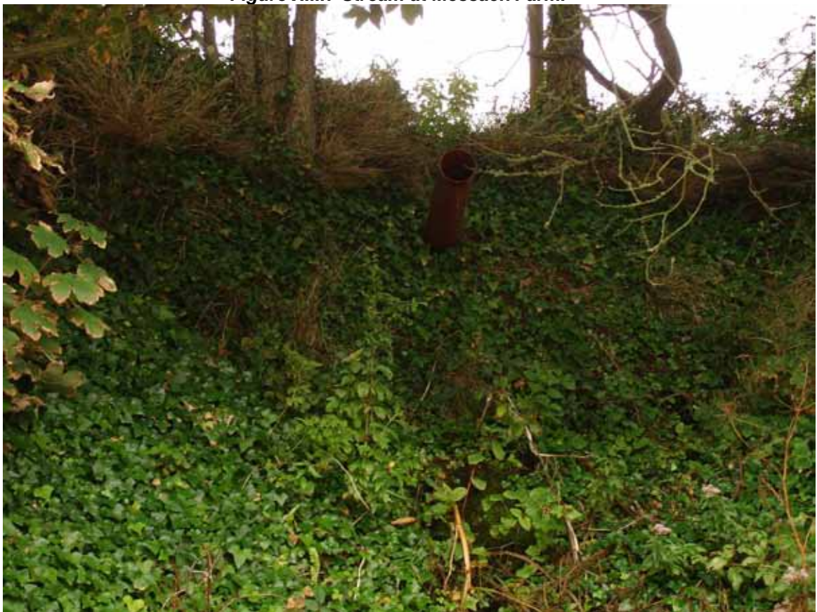
Figure XIII.8 Land drain pipe at St Just Pool.
