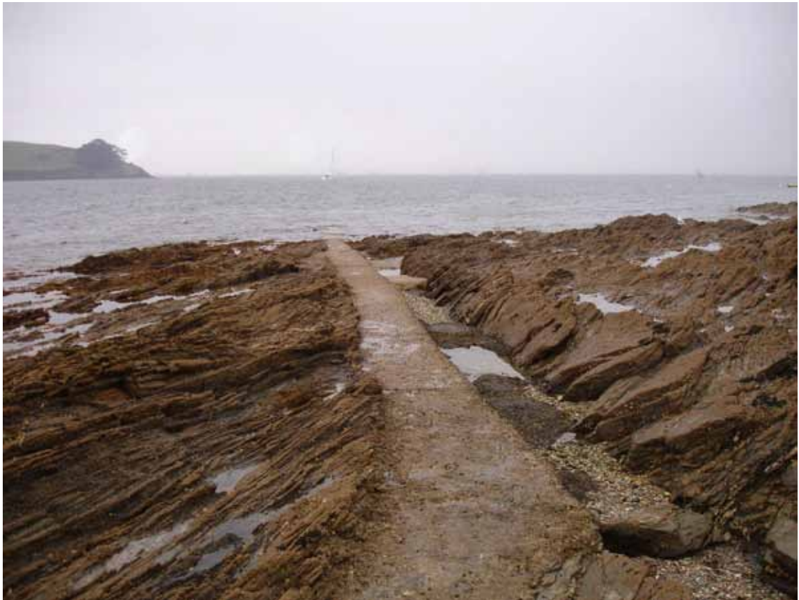
Figure XIII.15 St. Mawes PS No1 outfall.
