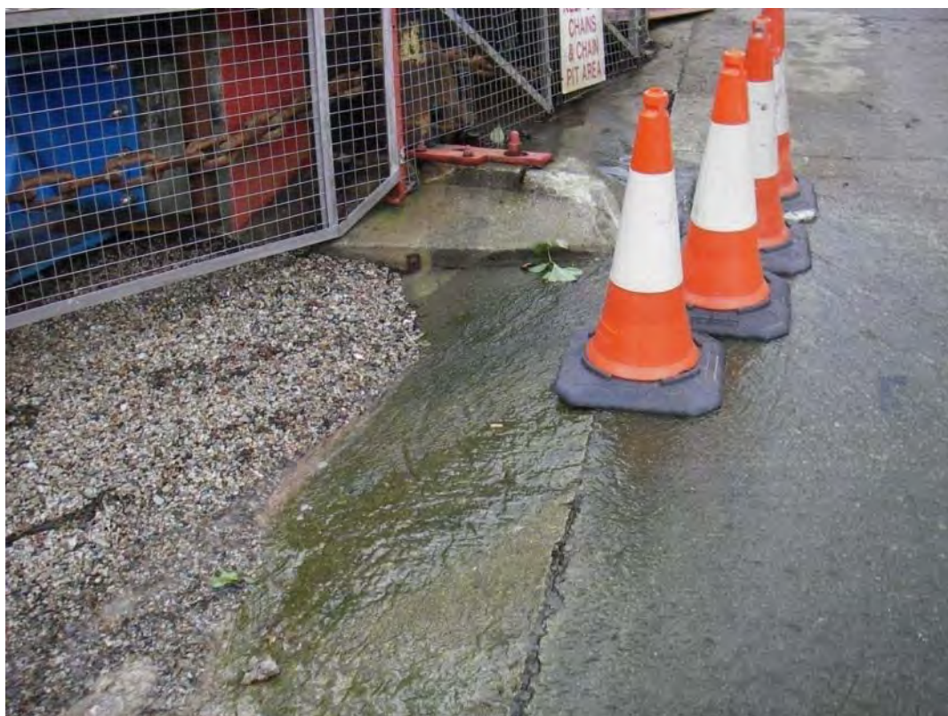
Figure 74. Stream outlet at King Harry Ferry slipway
