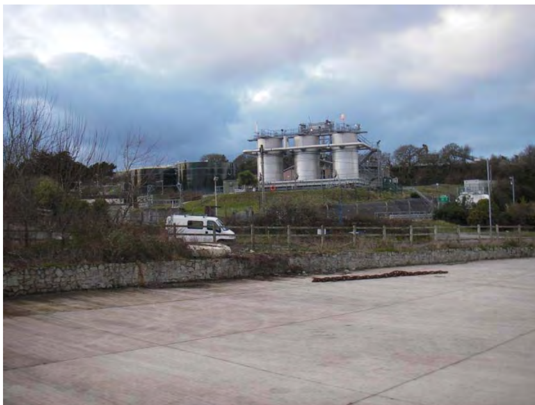
Figure 79. Newham Sewage Treatment Works, Truro
