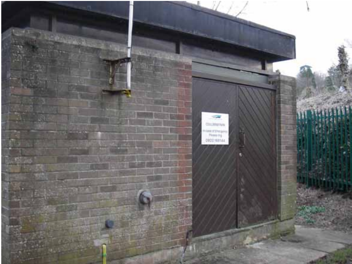
Figure XIII.10. Coulson Park Pumping Station.
