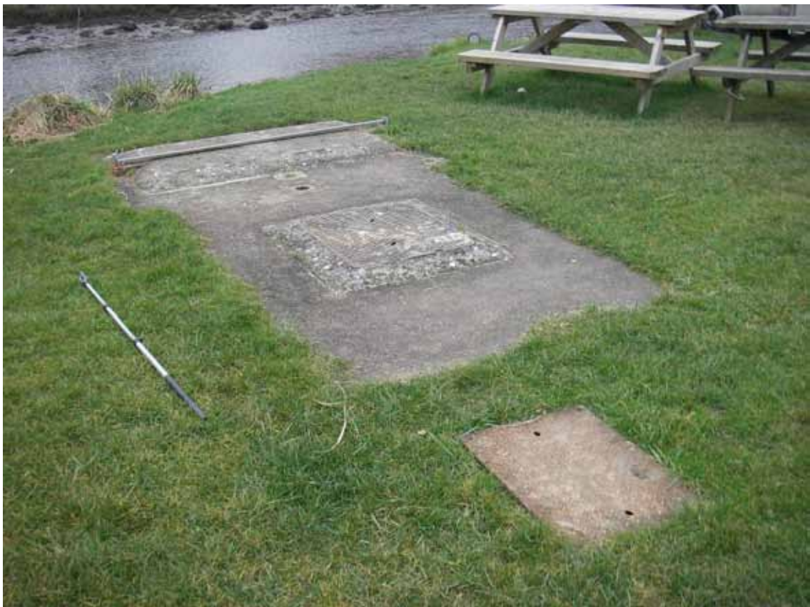
Figure A.15. Manhole covers at Lerryn.
