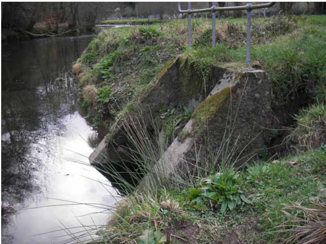
Figure XIII.11. Coulson Park Storm Outfall.
