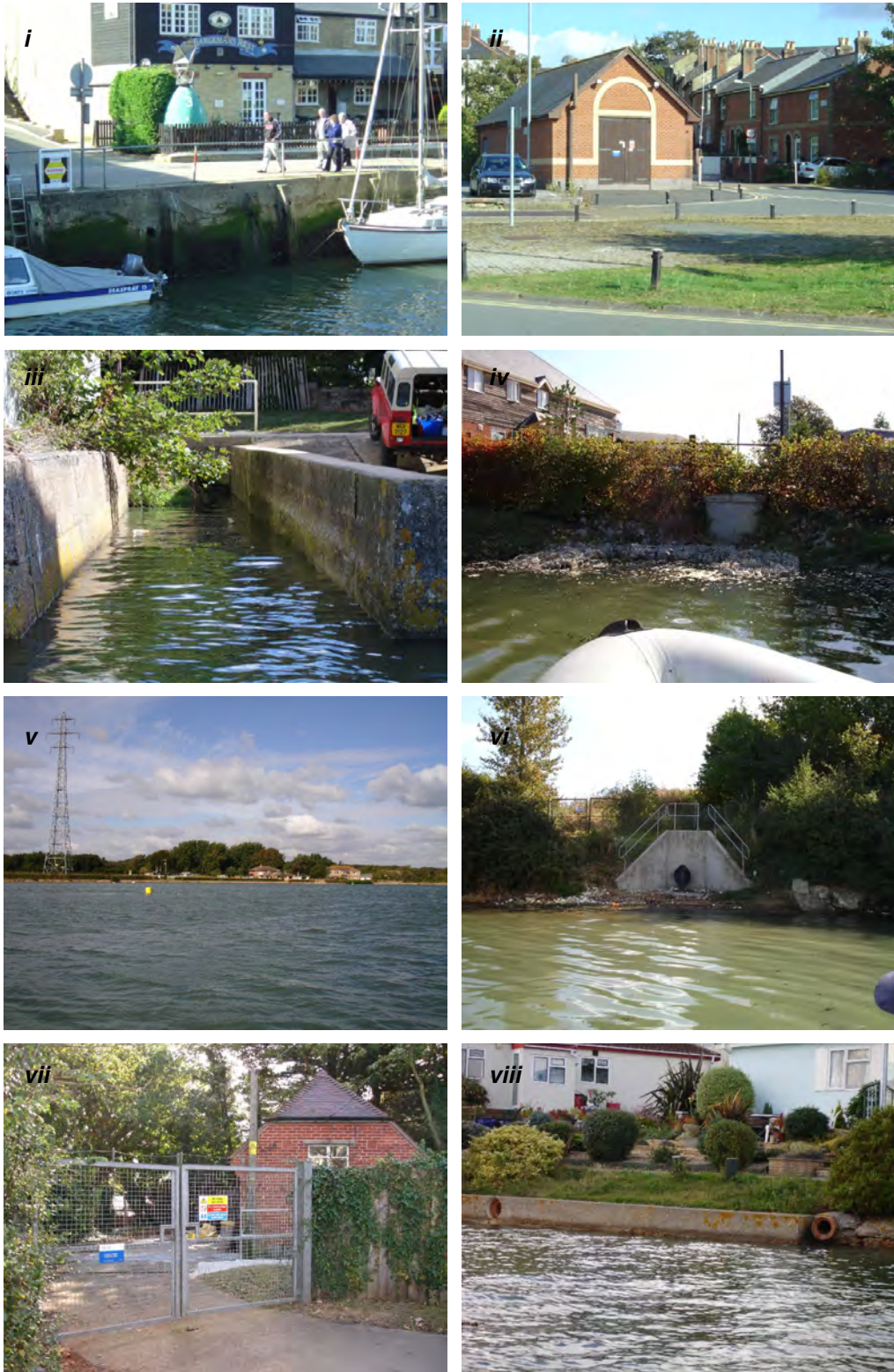
Figure A3: Photos of: i) discharge at Bargemans Rest public house, ii) Newport Quay sewage pumping station, iii) culverted stream at Seaclose Quay, iv) outfall from Newport sewage pumping station outfall at high water, v) Fairlee STW outfall buoy, vi) Fairlee transfer outfall, vii) Dodnor sewage pumping station, viii) Dodnor cottages.
