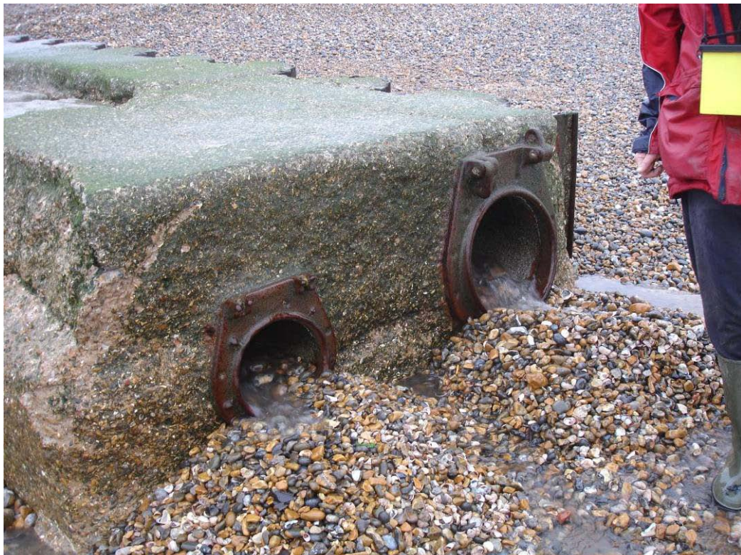
Figure XIII.29 Surface water outfalls
