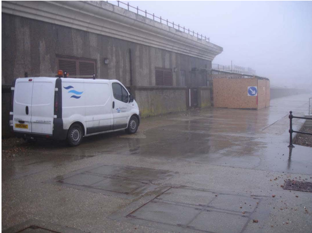
Figure XIII.28 Large pumping station
