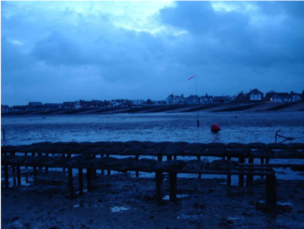
Figure XIII.14 Trestles at Whitstable
