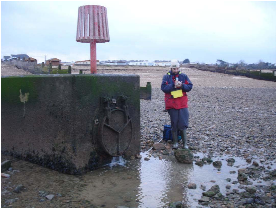
Figure XIII.17 Surface water outfall
