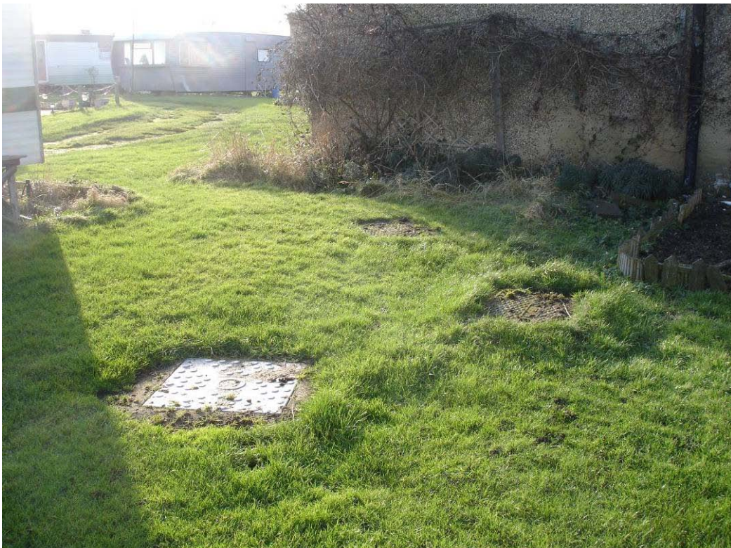
Figure XIII.23 Inspection covers possible associated with septic tank in caravan park
