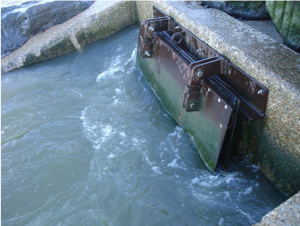
Figure XIII.12 Surface water outfall
