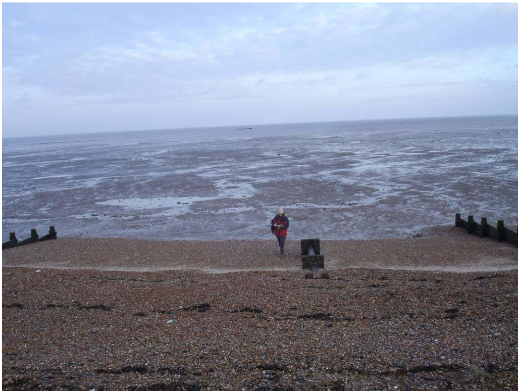
Figure XIII.19 Surface water outfall
