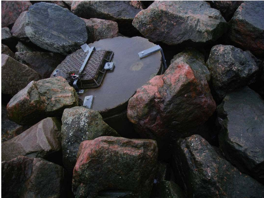
Figure XIII.30 Inspection cover by Hampton Pier
