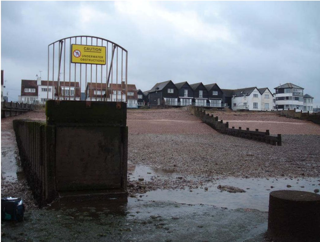
Figure XIII.16 Surface water outfall
