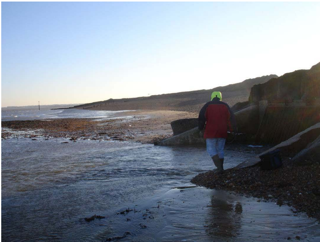
Figure XIII.11 Surface water outfall near Reculver
