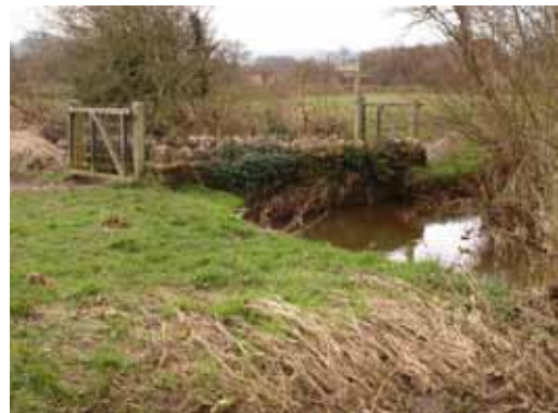
Photo 6: Corfe River at Sharford Bridge
