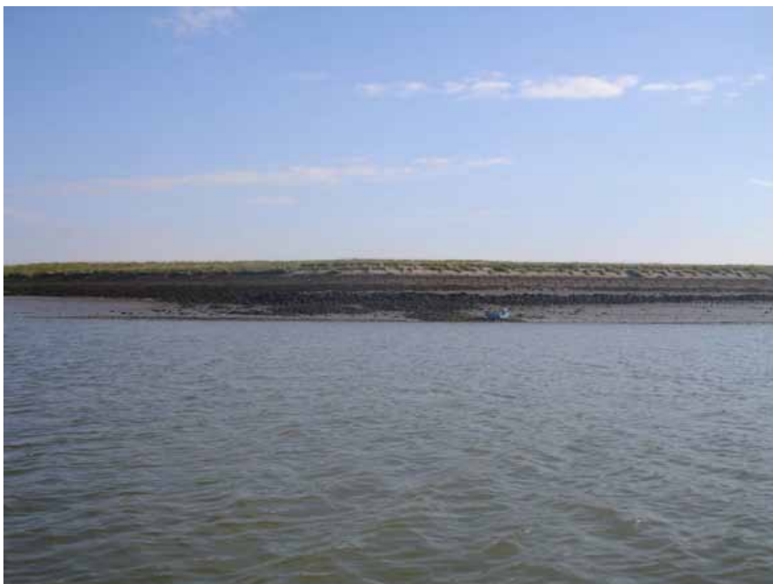
Figure XIII.6 - End of line of trestles along low water mark, Wallasea Island shore, R. Roach
