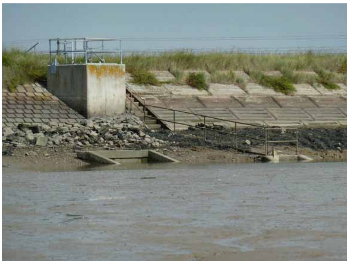
Figure XIII.9 - Rochford STW outfall
