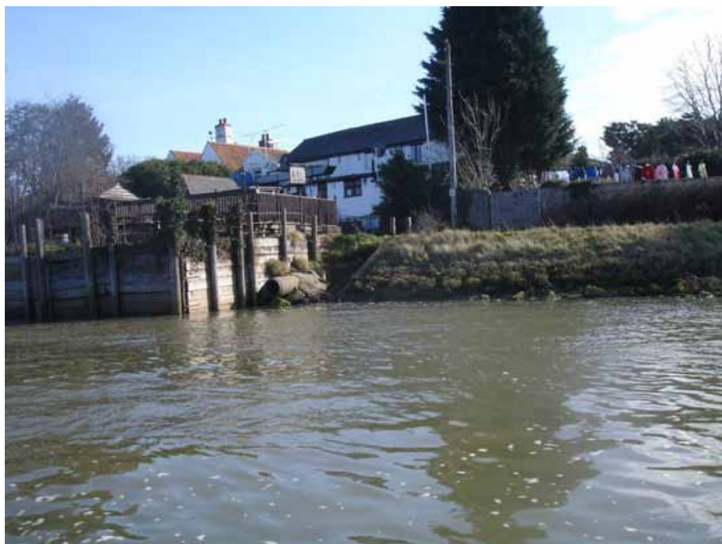
Figure XIV.8 Concrete pipe, Brandy Hole Reach
