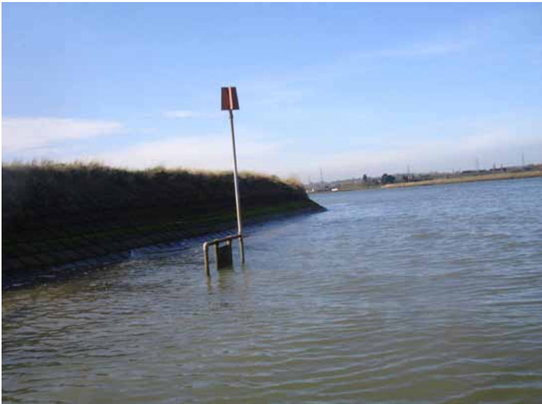
Figure XIV.6 Intermittent sewage outfall marker post
