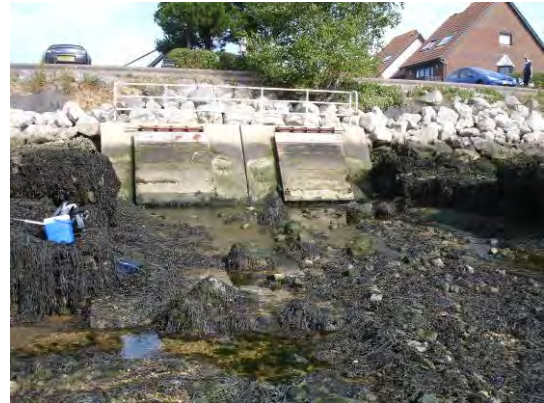
4: Hythe Village Marina sluice
