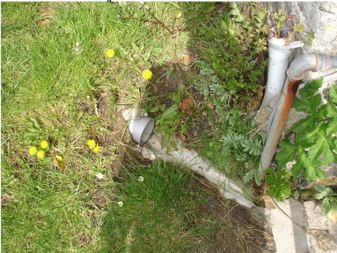
Figure XIII.9 PVC pipe from Porthpean Sailing Club
