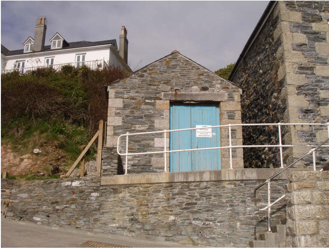
Figure XIII.4 Porthpean Pumping Station entrance.
