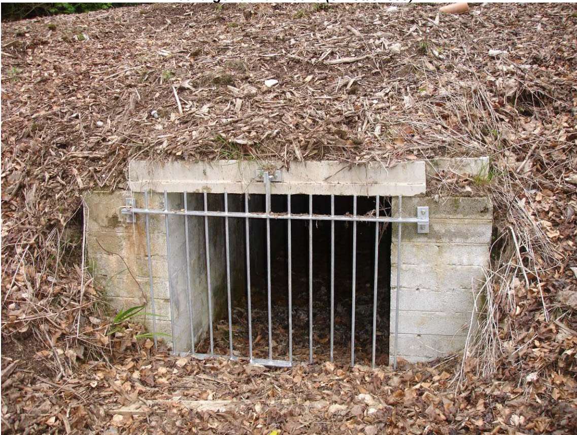
Figure XIII.13 Culvert at Duporth woodland south of new Holiday Village (03157/51197).
