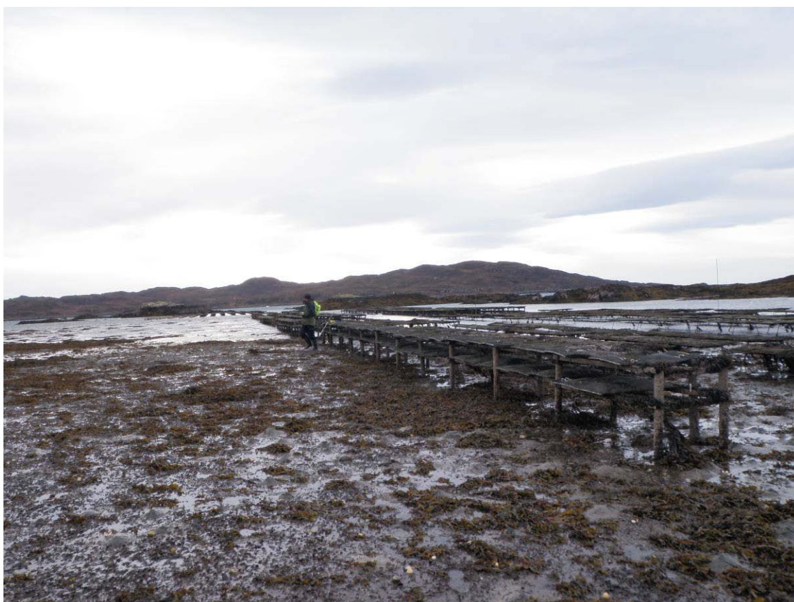
Figure 9 Trestles at Sgier Philip
