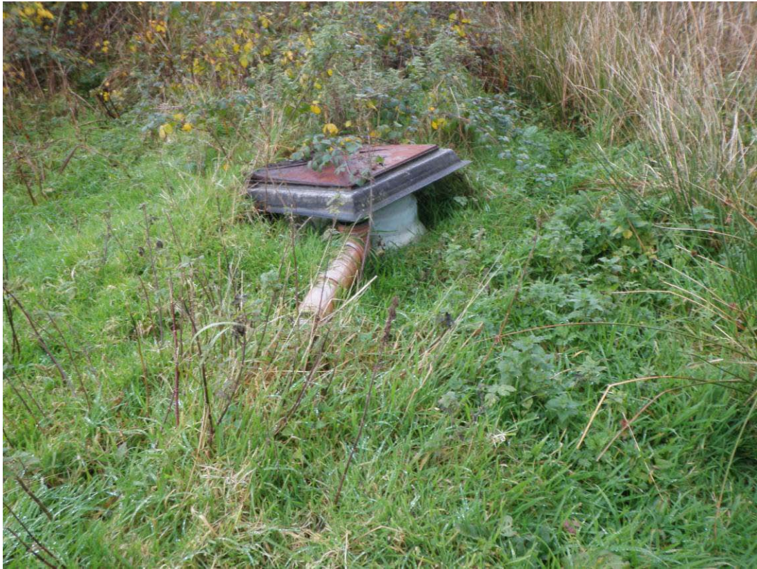
Figure 16. Septic tank with overflow pipe, Camas an t-Salainn
