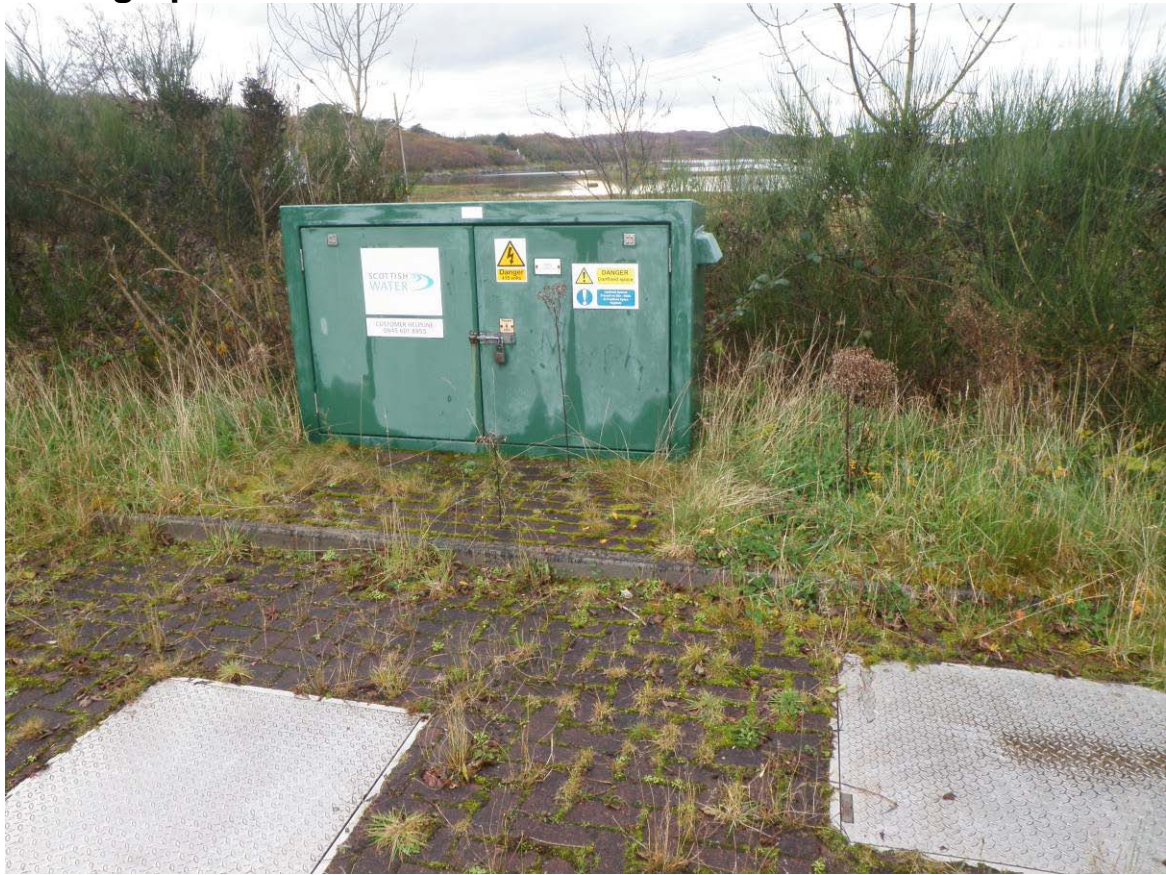
Figure 4 Septic tank at Arisaig
