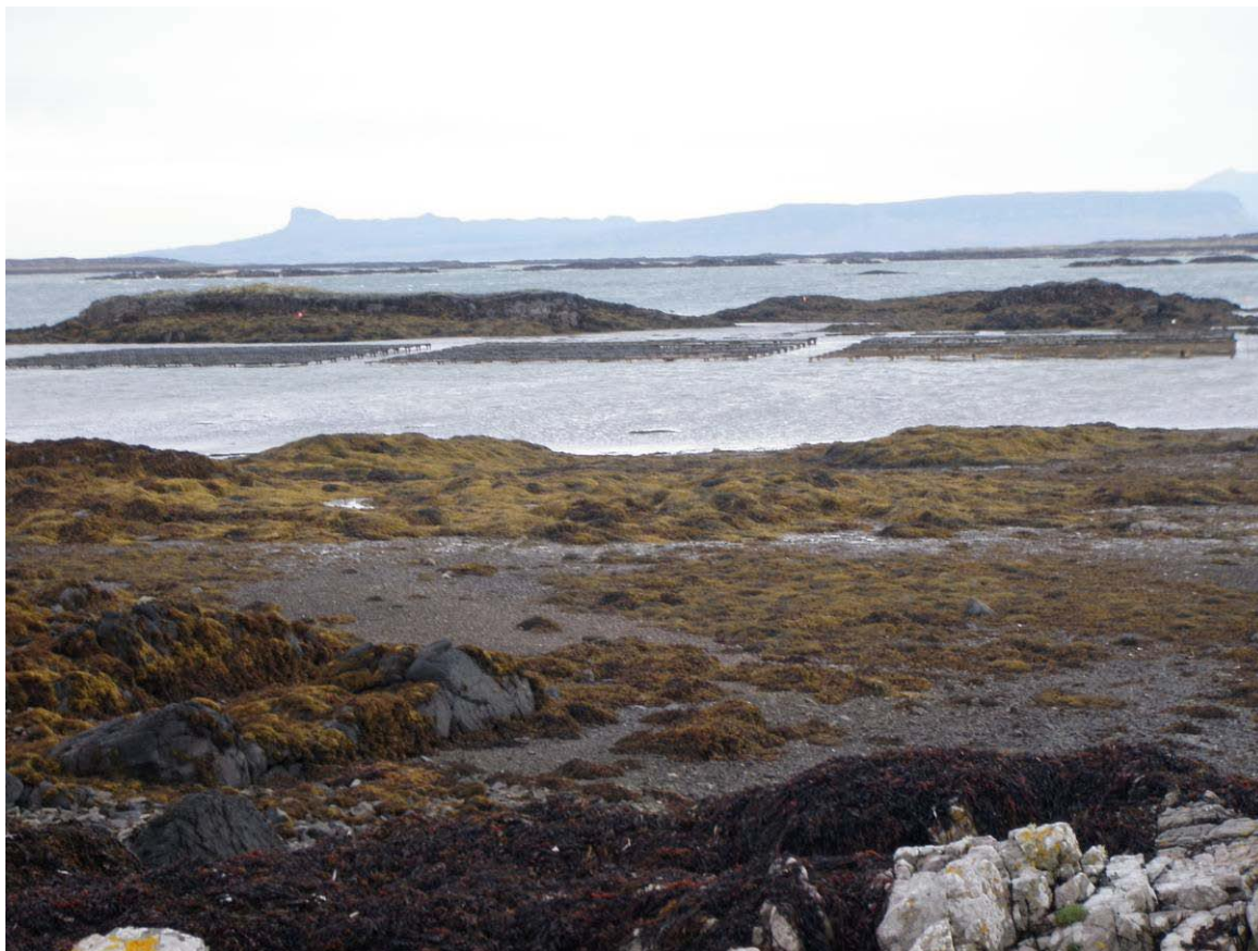
Figure 8 Overview of trestles near Sgeir Philip/North Channel
