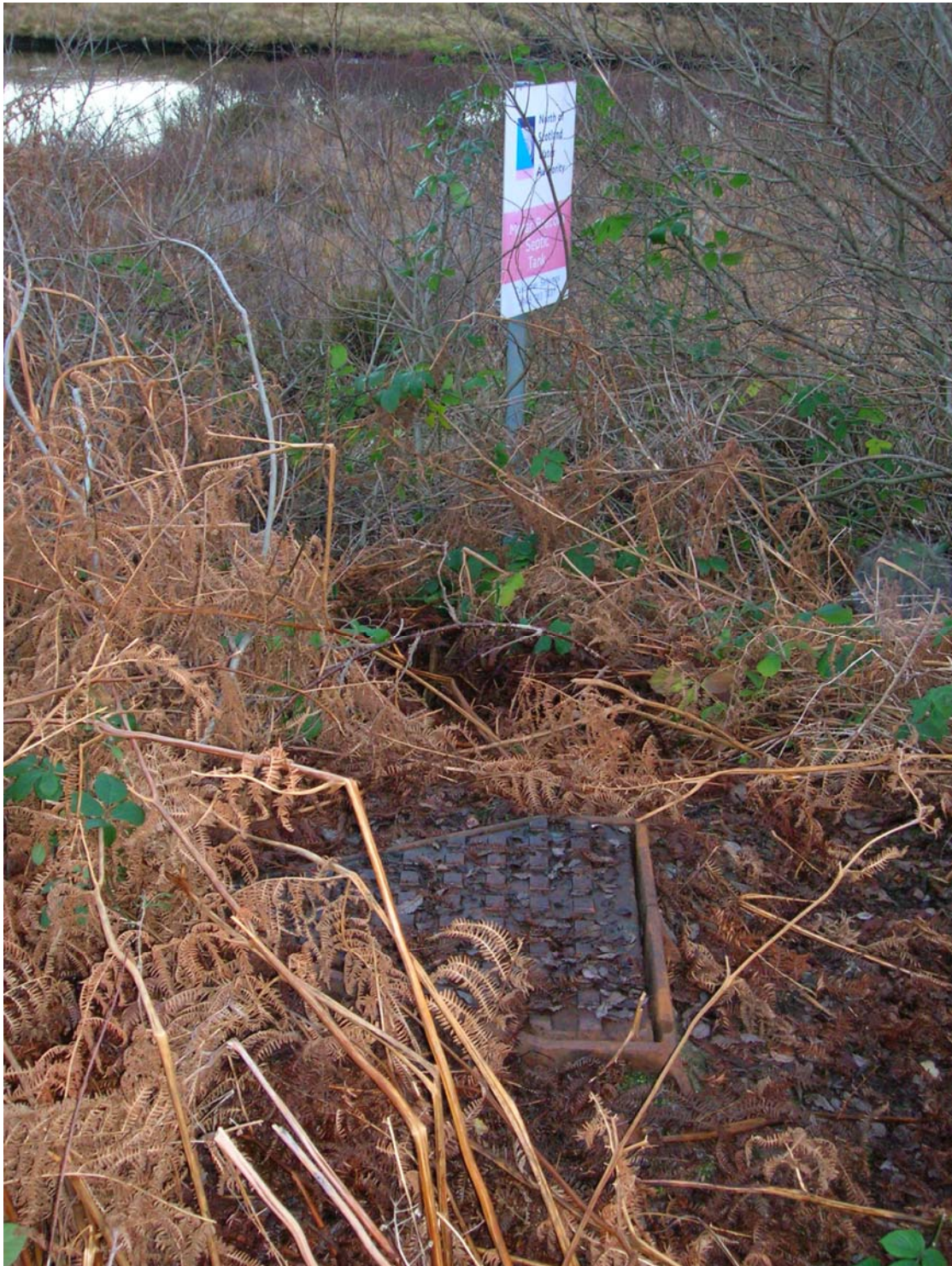
Figure 17. Morar/Bracora septic tank
