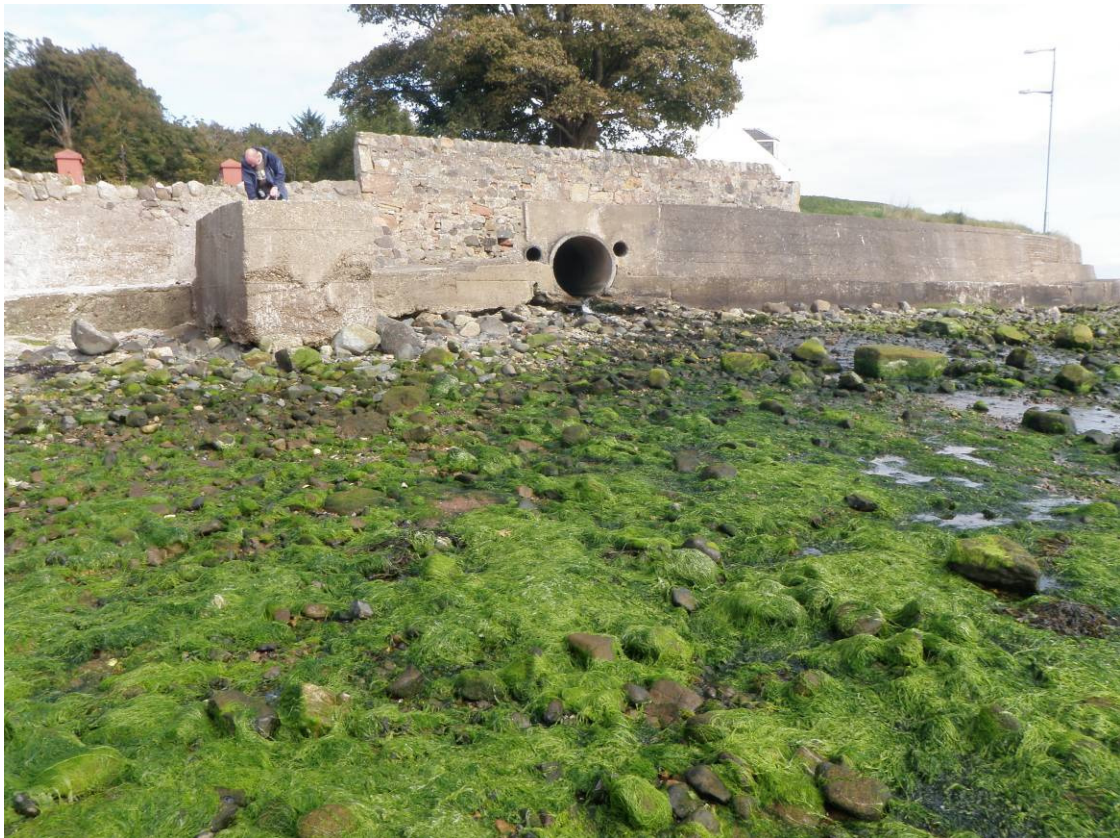
Figure 13. Stream through culvert, inspection covers, water sample 9
