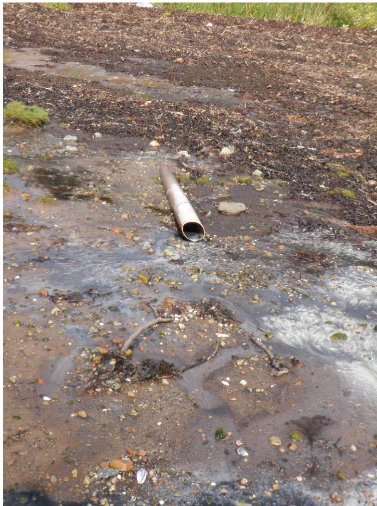
Figure 11. Pipe with sewage fungus on shoreline below, water sample 8
