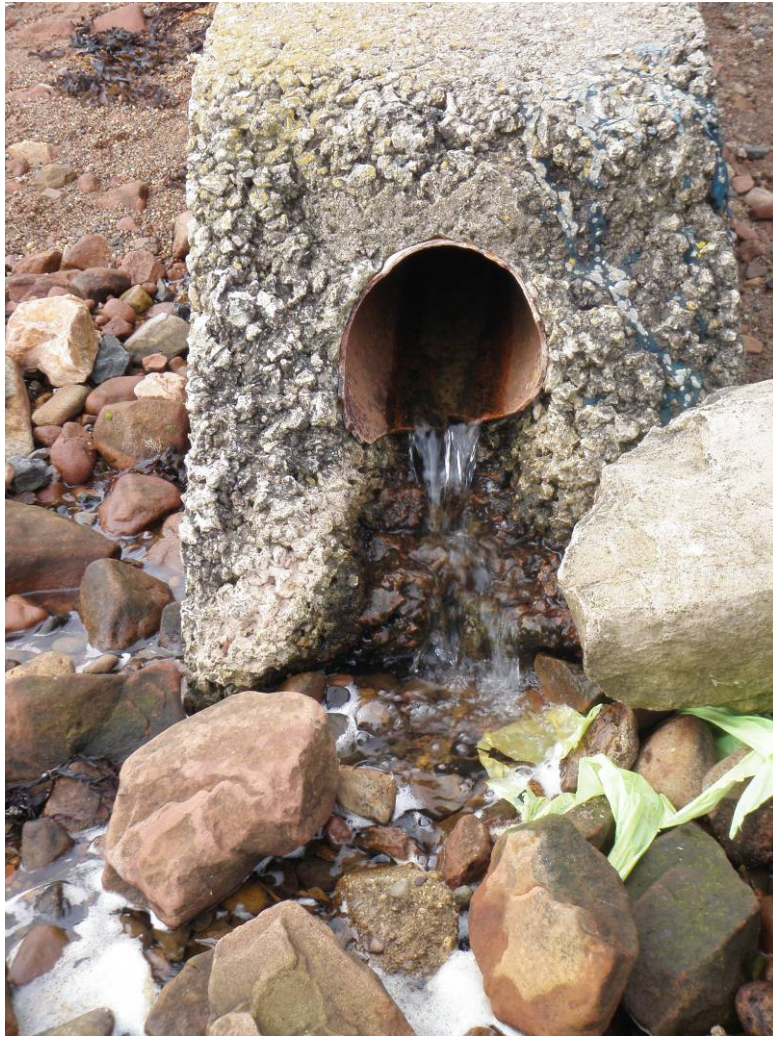
Figure 15. Pipe encased in concrete, large flow, water sample 13
