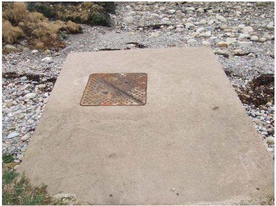
Figure 41. Concrete block with inspection cover, no visible outfall pipe
