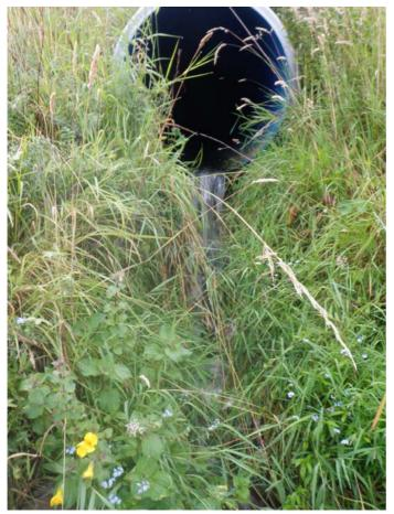
Figure 13. Flow through corrugated pipe in hillside below campground
