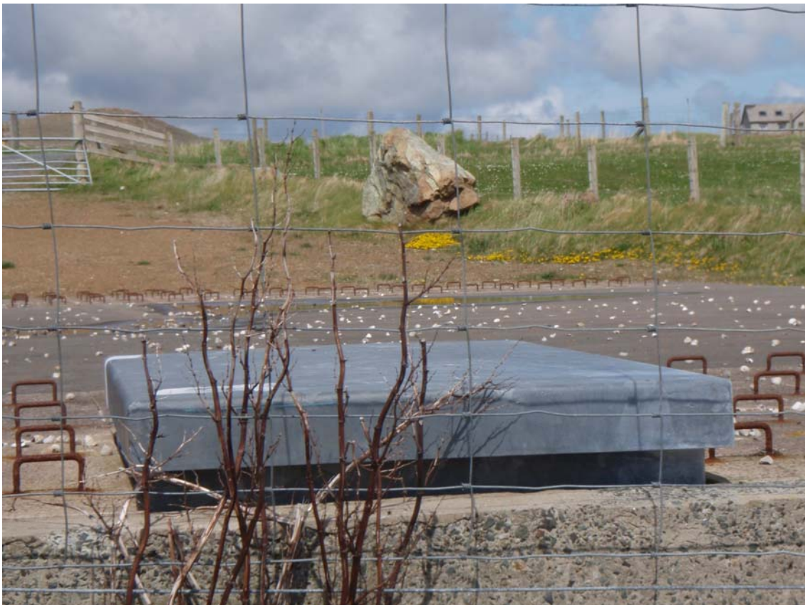
Figure 7. Scottish Water septic tank
