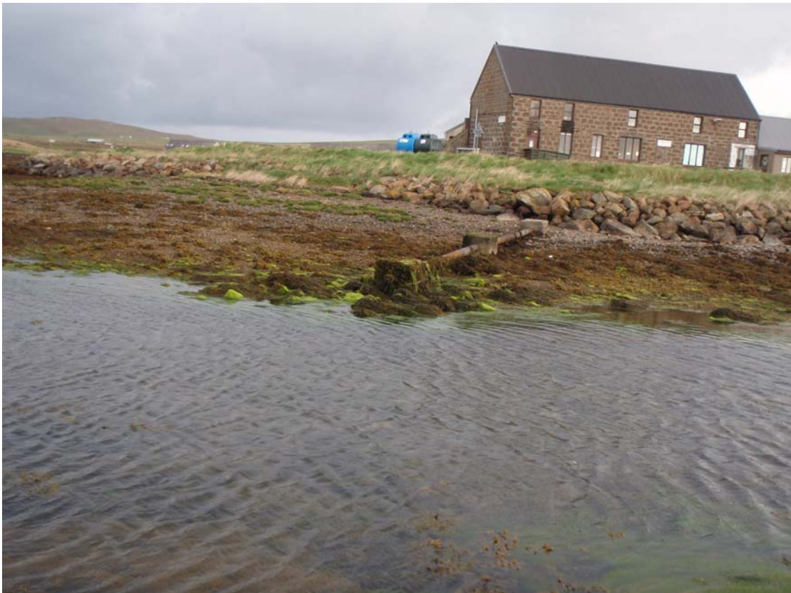
Figure 11. Scottish water emergency overflow
