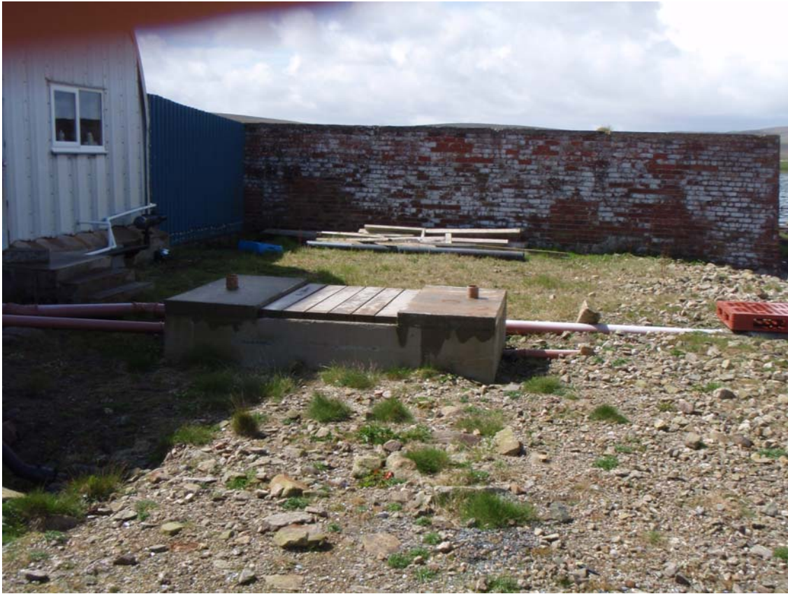
Figure 14. Septic tank at mussel shed
