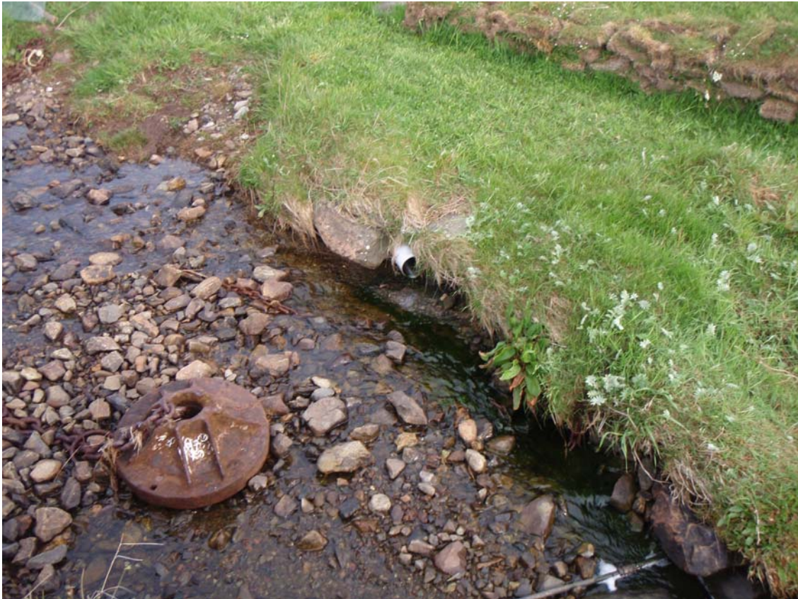
Figure 12. Septic tank discharge to stream which flows toward trestles
