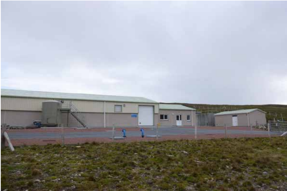
Figure 12 – Yell Water Treatment Works
