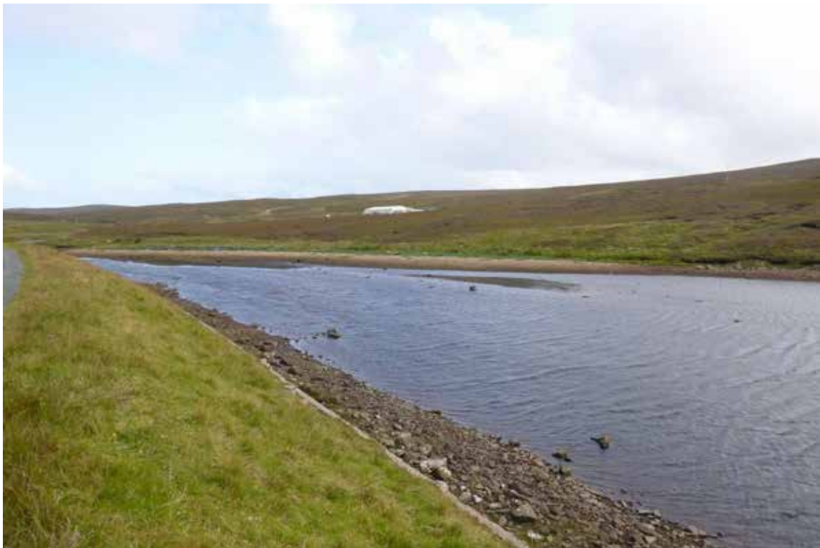
Figure 15 – Pool at the Burn of Gossawater inshore from the culvert.
