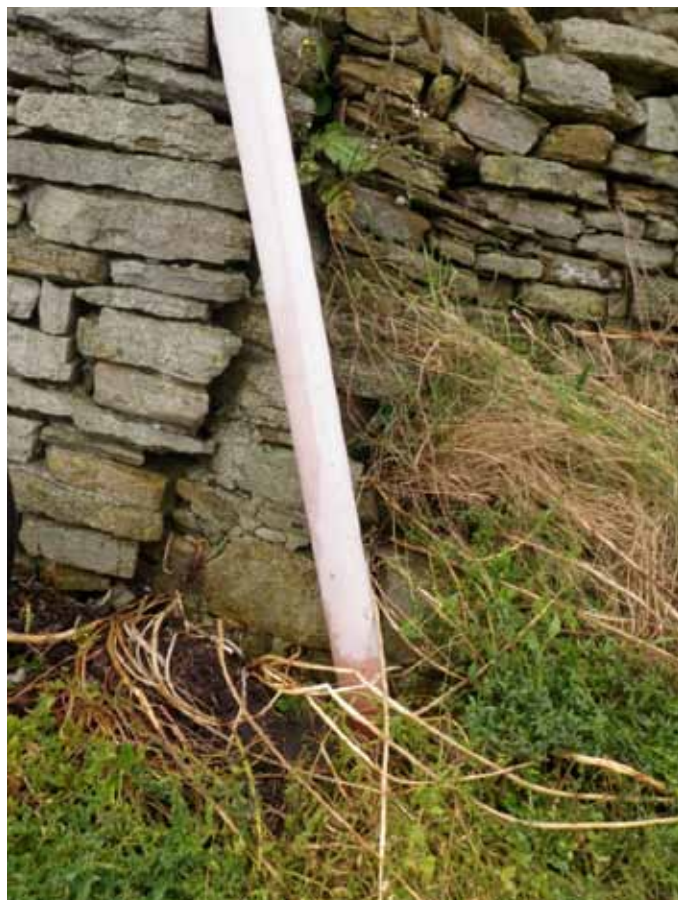
Figure 6. Plastic pipe to ground at upper shore
