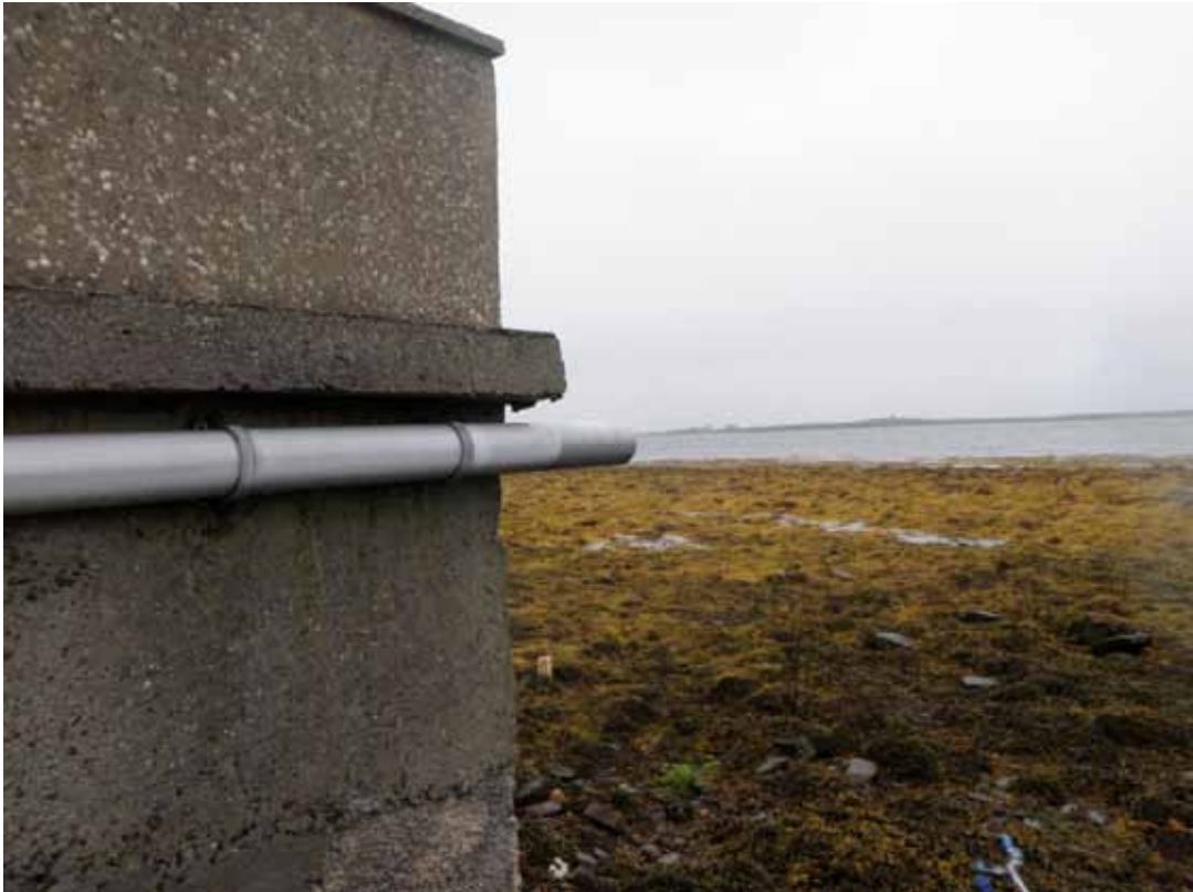
Figure 5. New drainage pipe along seawall at Kettletoft.
