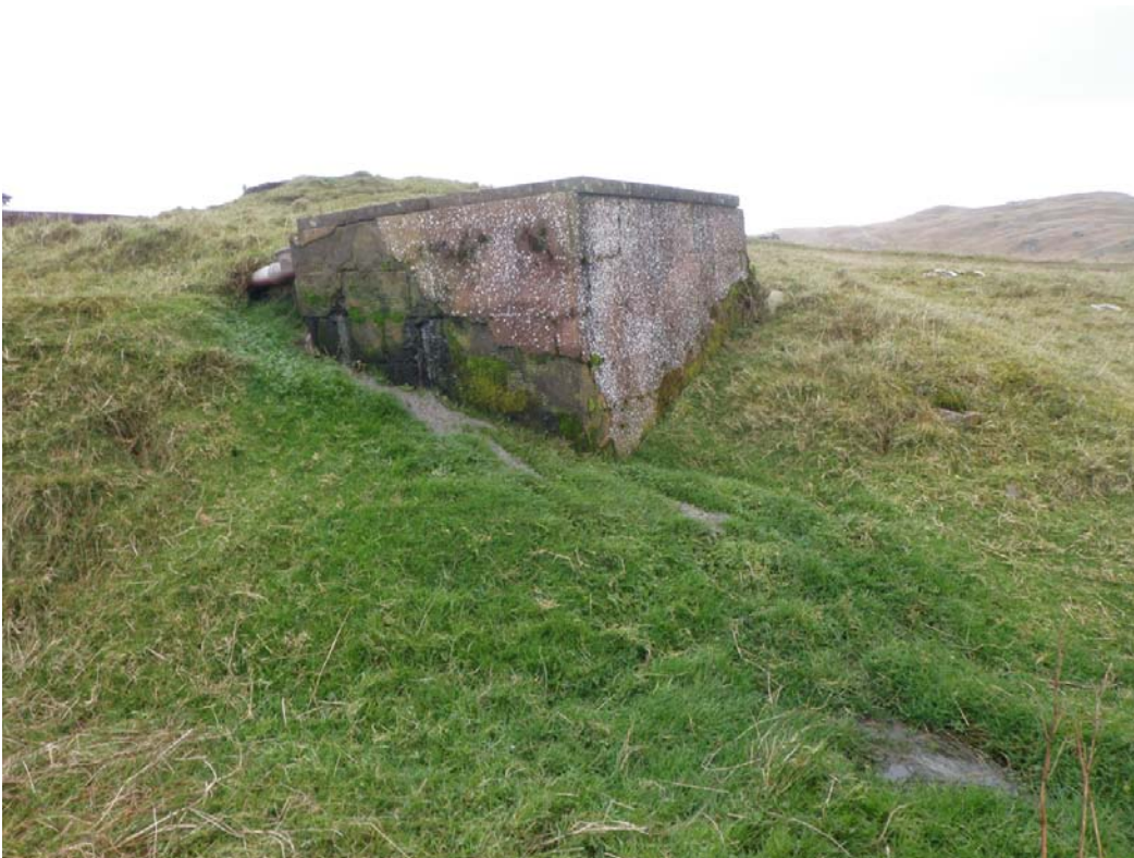
Figure 8 – Septic tank at Biggins
