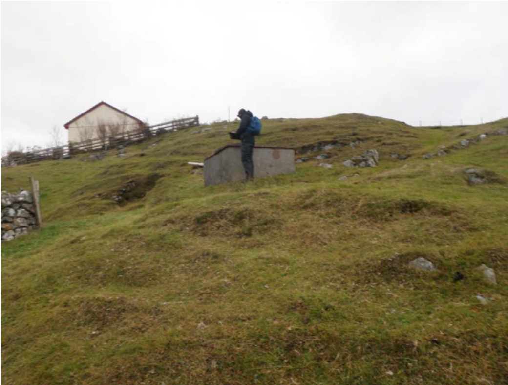
Figure 17 – Septic tank at the last house on the western shore.
