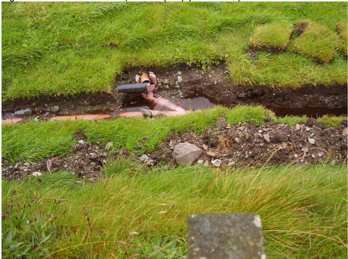
Figure 29. Busta060921. Exposed septic pipe under repair.
