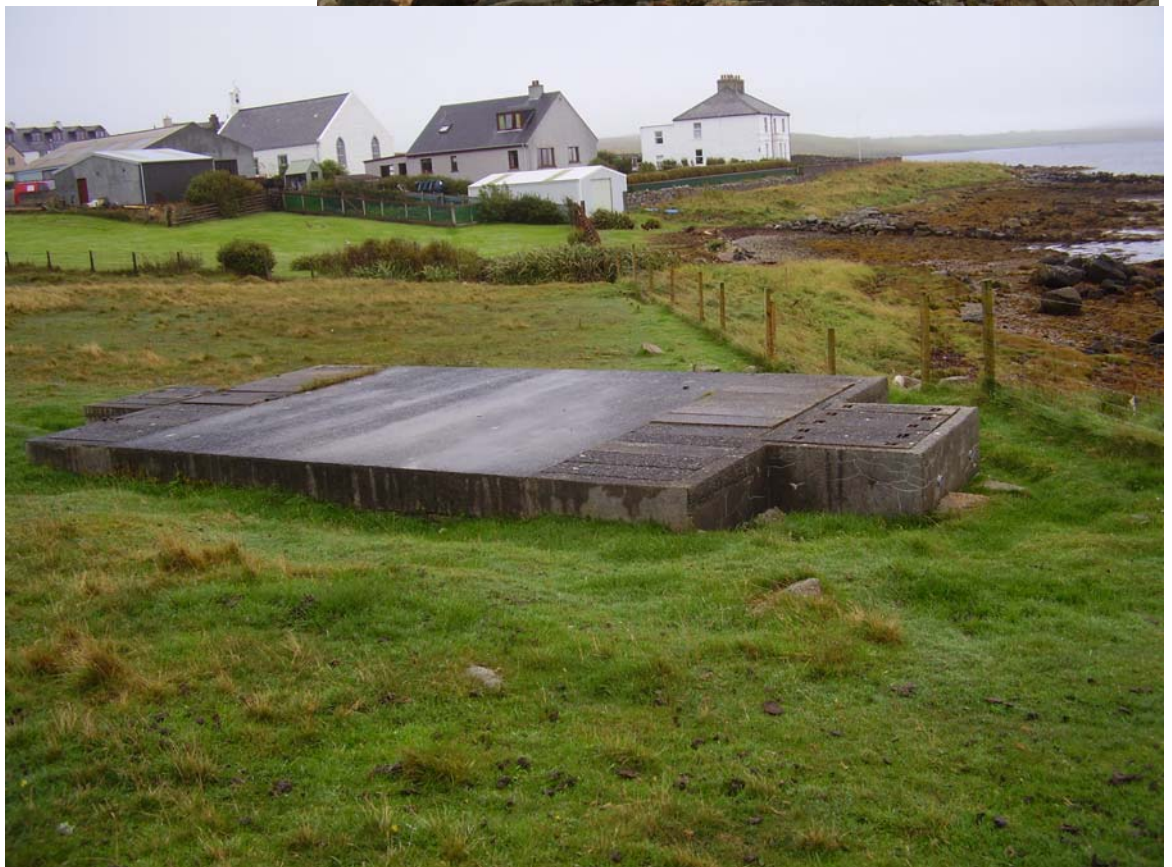
Figure 19. Busta060903. Another big septic tank.
