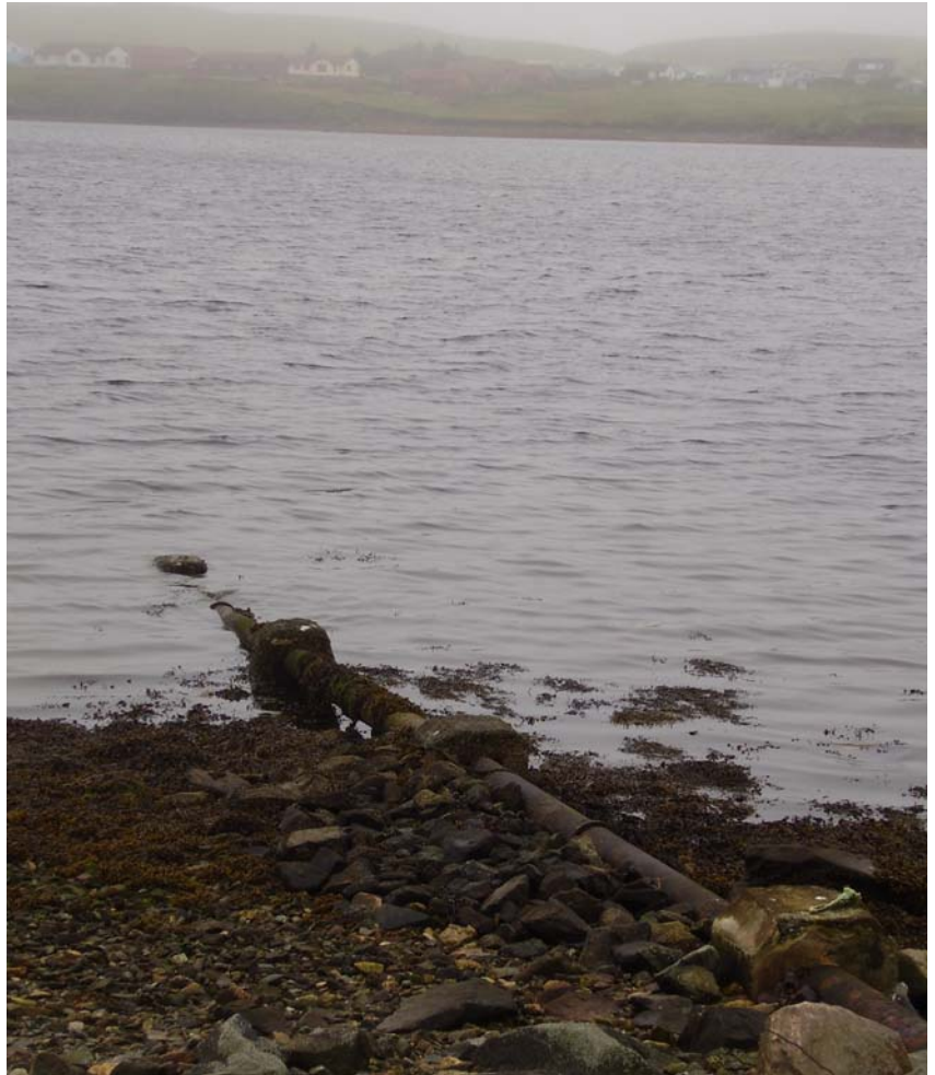
Figure 18. Busta060902. Discharge pipe for tank.
