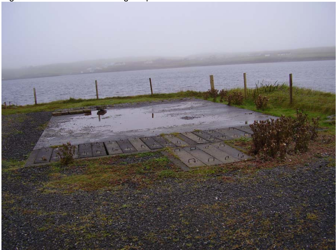
Figure 17. Busta060901. Large septic tank cover.
