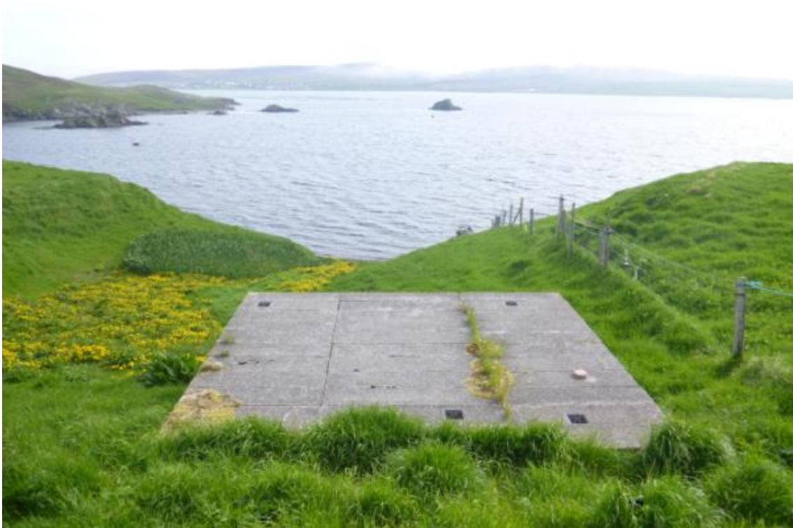
Figure 15 – Septic tank south of the Muckle Roe bridge.
