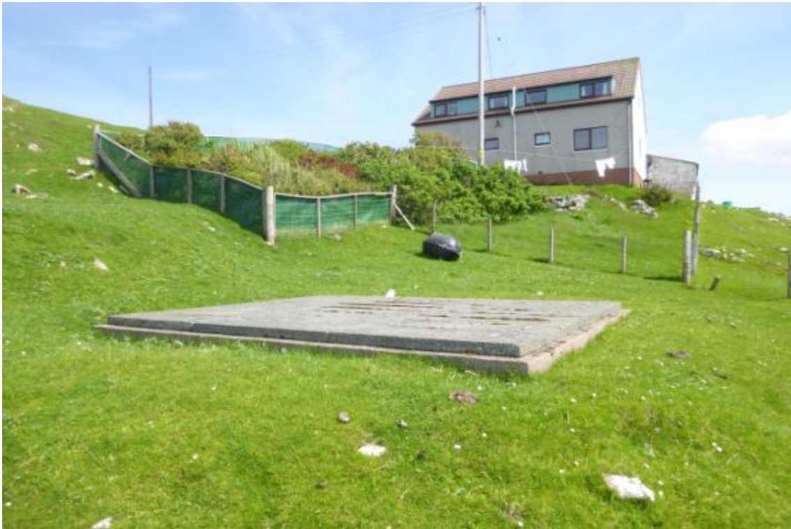
Figure 14 – Septic tank servicing a house at Wetherstanes.
