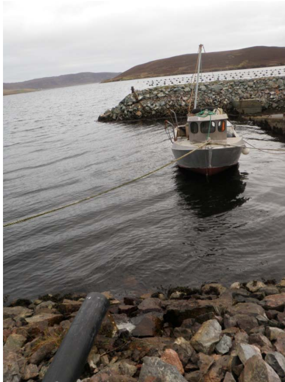
Figure 14 – Land drainage pipe discharging to jetty adjacent to the Greentaing fishery.
