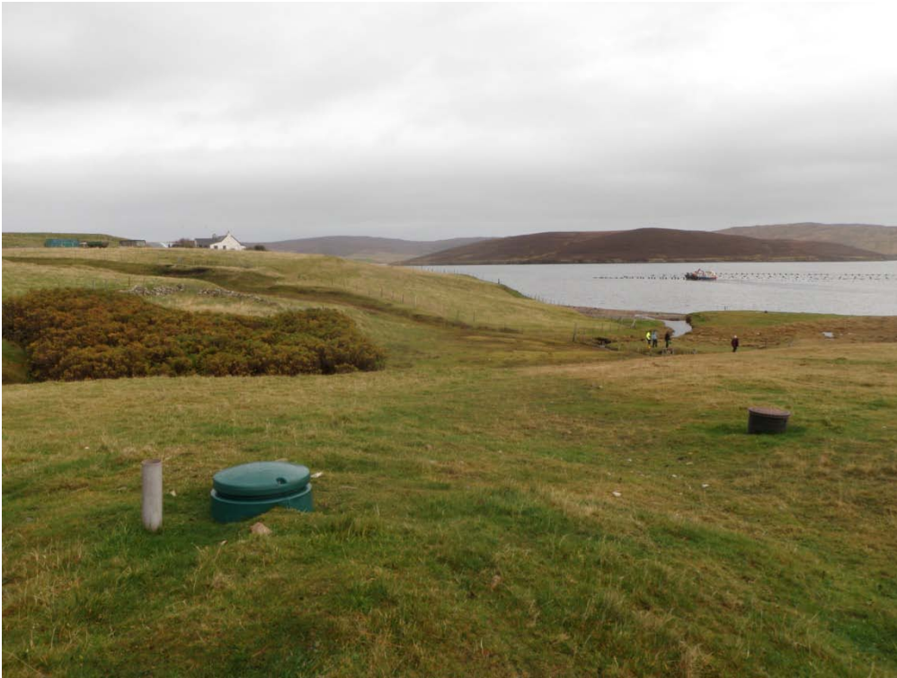
Figure 10 – Septic tank below an occupied property adjacent to the Buddascord fishery.
