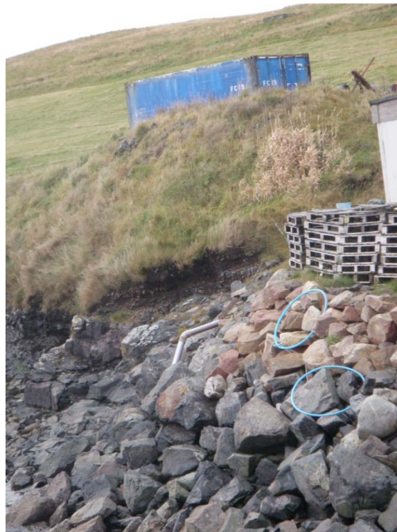
Figure 13 – Discharge pipe from portacabin at the jetty near the Greentaing fishery.
