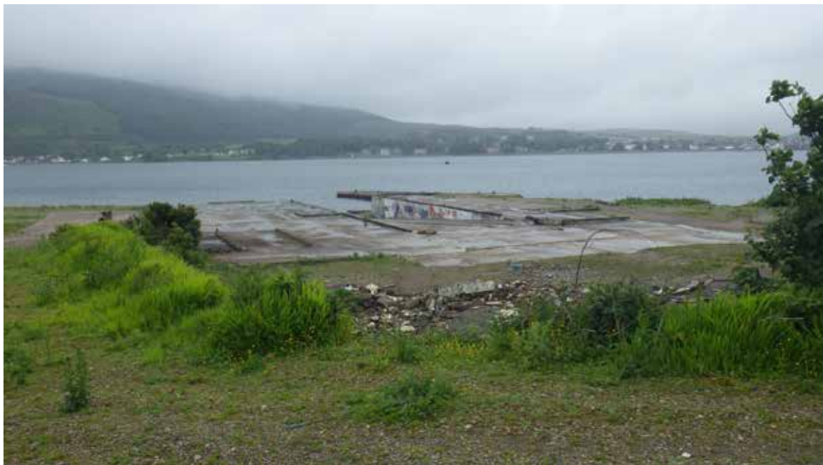
Figure 4: Overview of the abandoned site of the Campbeltown boatyard, looking SW across Campbeltown Loch (Waypoint 12)
