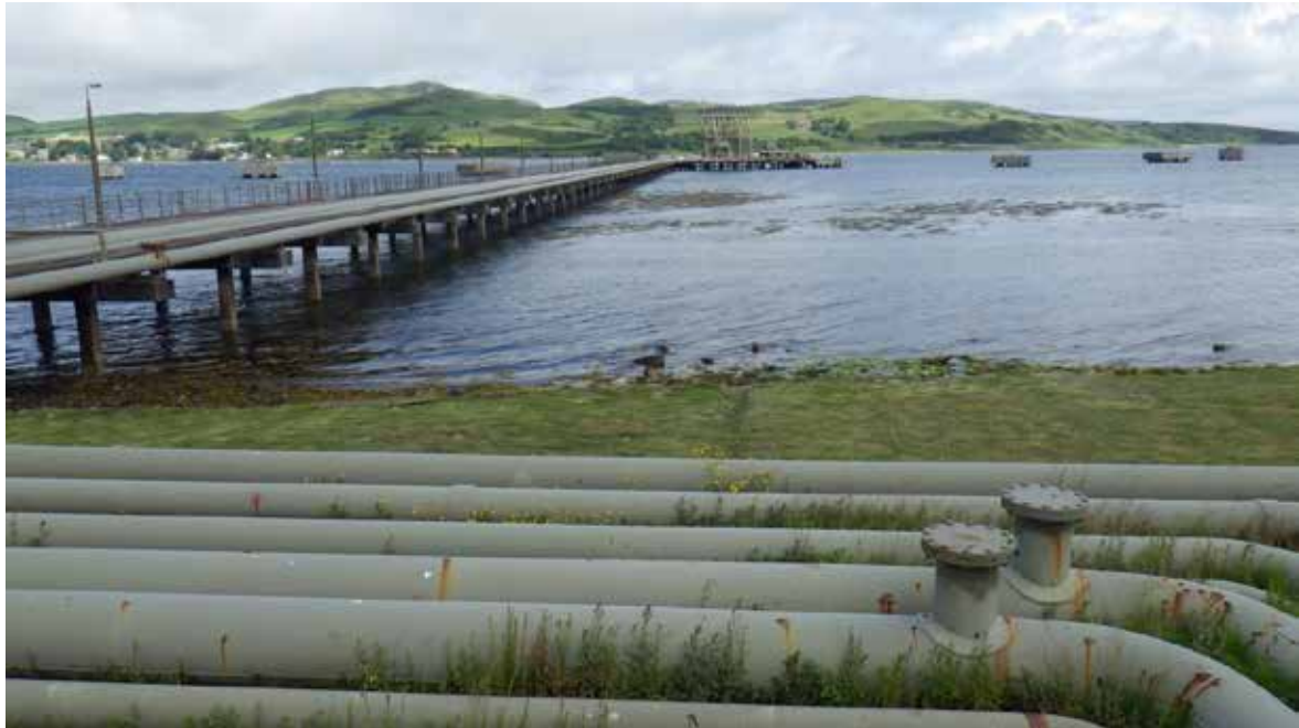
Figure 17: NATO refuelling Pier. (Waypoint 63)
