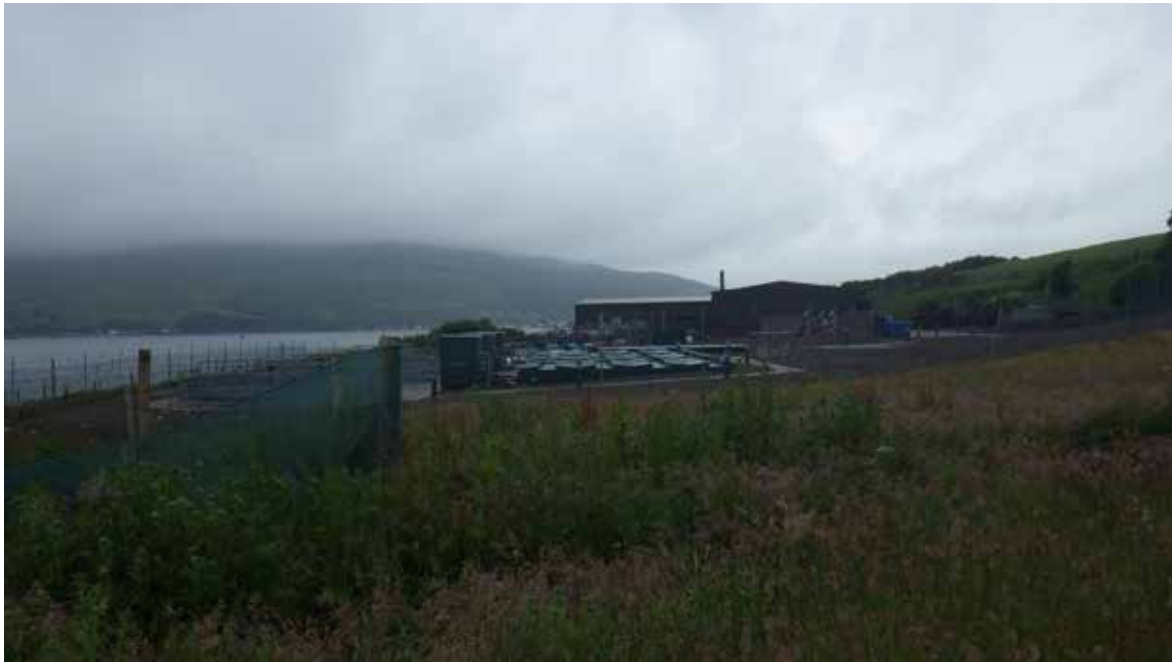
Figure 3: Overview of Slaty Farlan WWTW, looking west (Waypoint 4)
