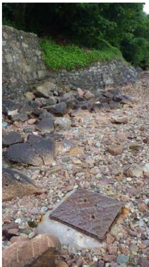
Figure 14: Manhole on inter-tidal shore in village of Kilkerran. (Waypoint 46)
