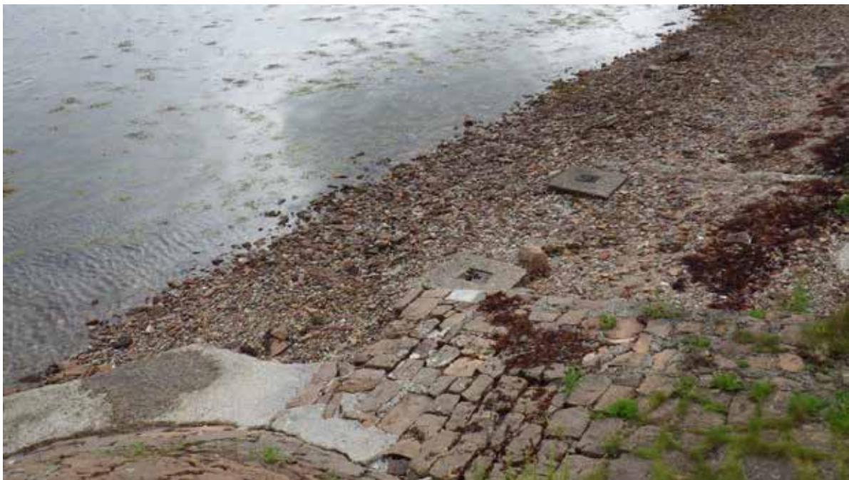
Figure 12: Small manholes at SE end of esplanade. (Waypoint 42)
