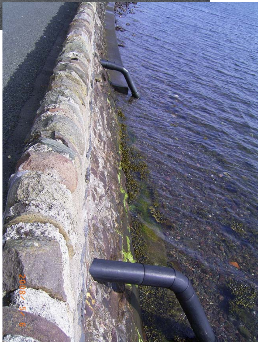
Figure 8. Black pipes to main sewage pipeline
