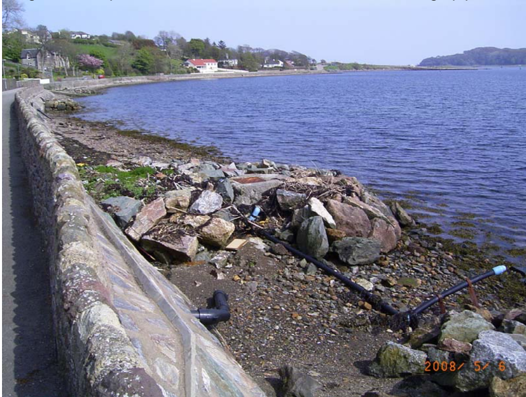
Figure 9. Inspection cover with vent on north shore sewage pipeline
