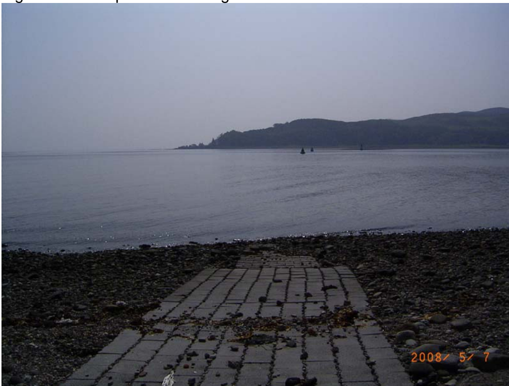
Figure 12. Campbeltown sewage works outfall
