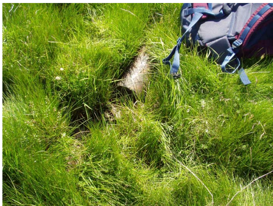
Figure 9. 6" clay pipe below house
