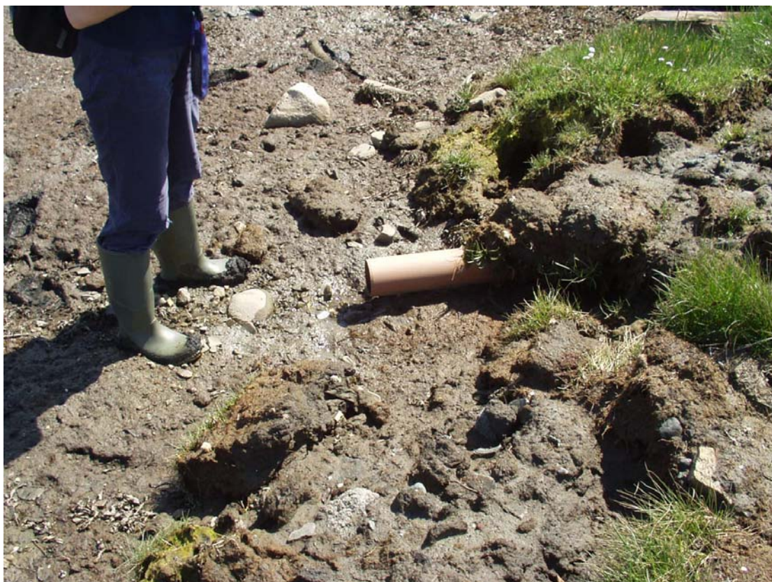
Figure 10. 4" plastic pipe down to shore, dripping, no smell
