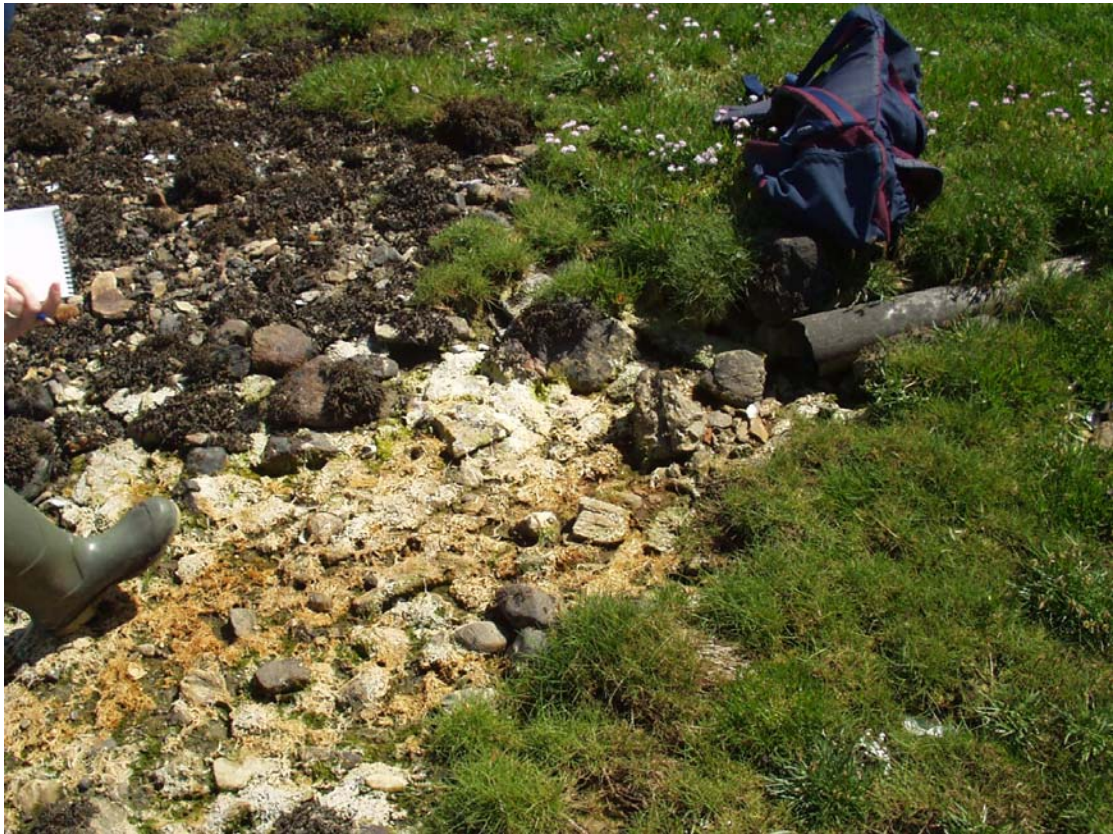
Figure 12. 6" cast iron pipe, not flowing
