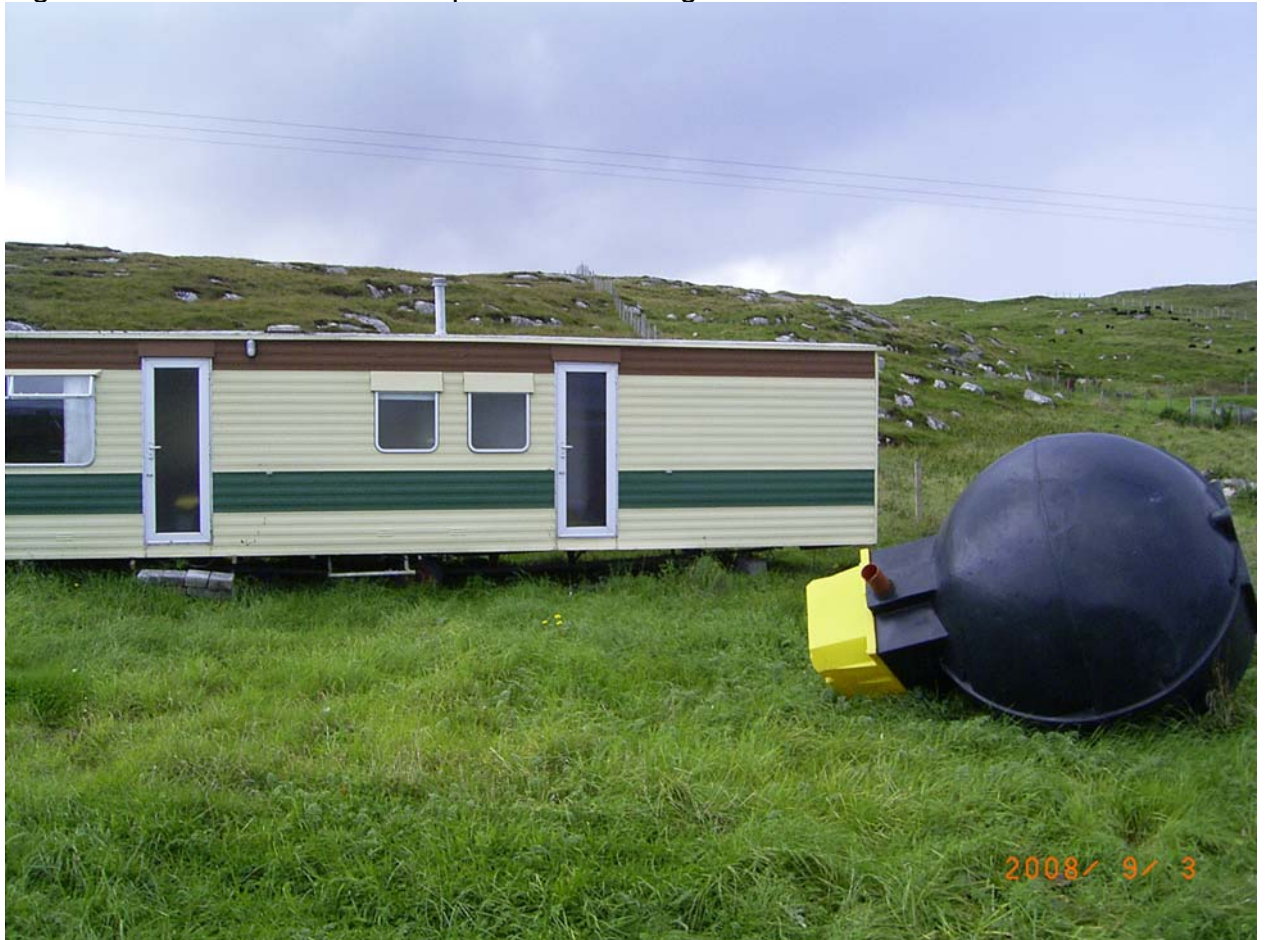
Figure 7 Static caravan with septic tank awaiting installment
