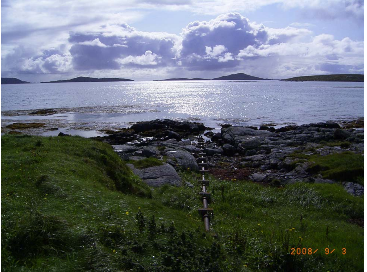
Figure 4 Public toilet discharge pipe
