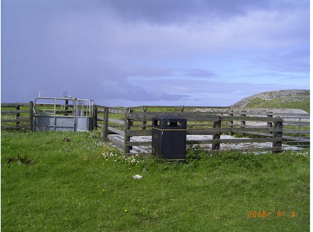
Figure 6 Concrete livestock pen
