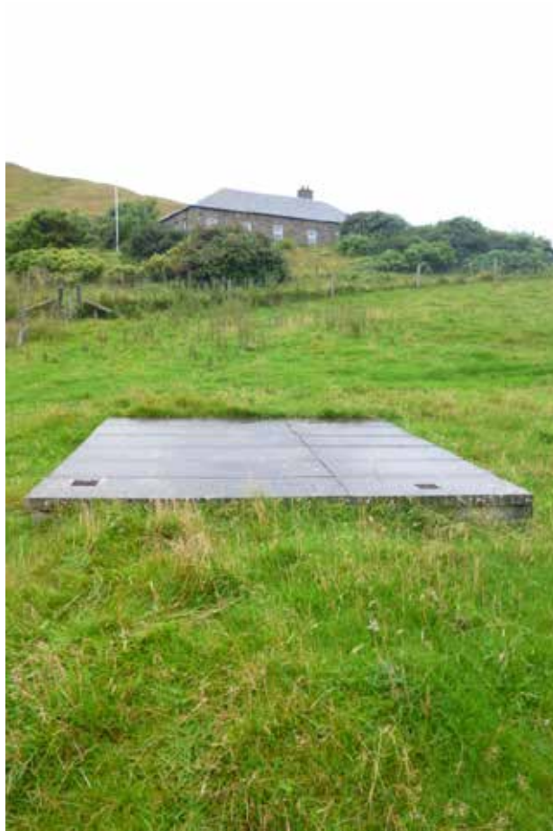
Figure 10 – Concrete septic tank servicing houses in the Wester Quarff area.
