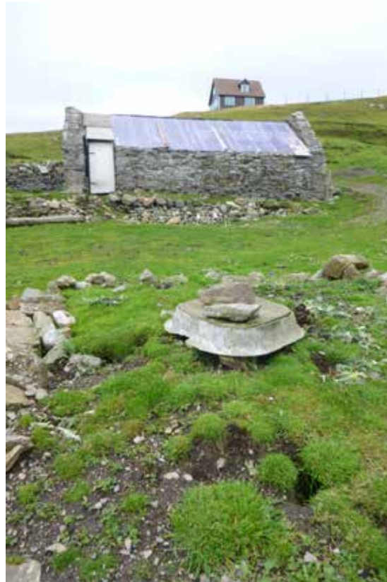
Figure 13 – Septic tank servicing two houses in the East Hogaland area.
