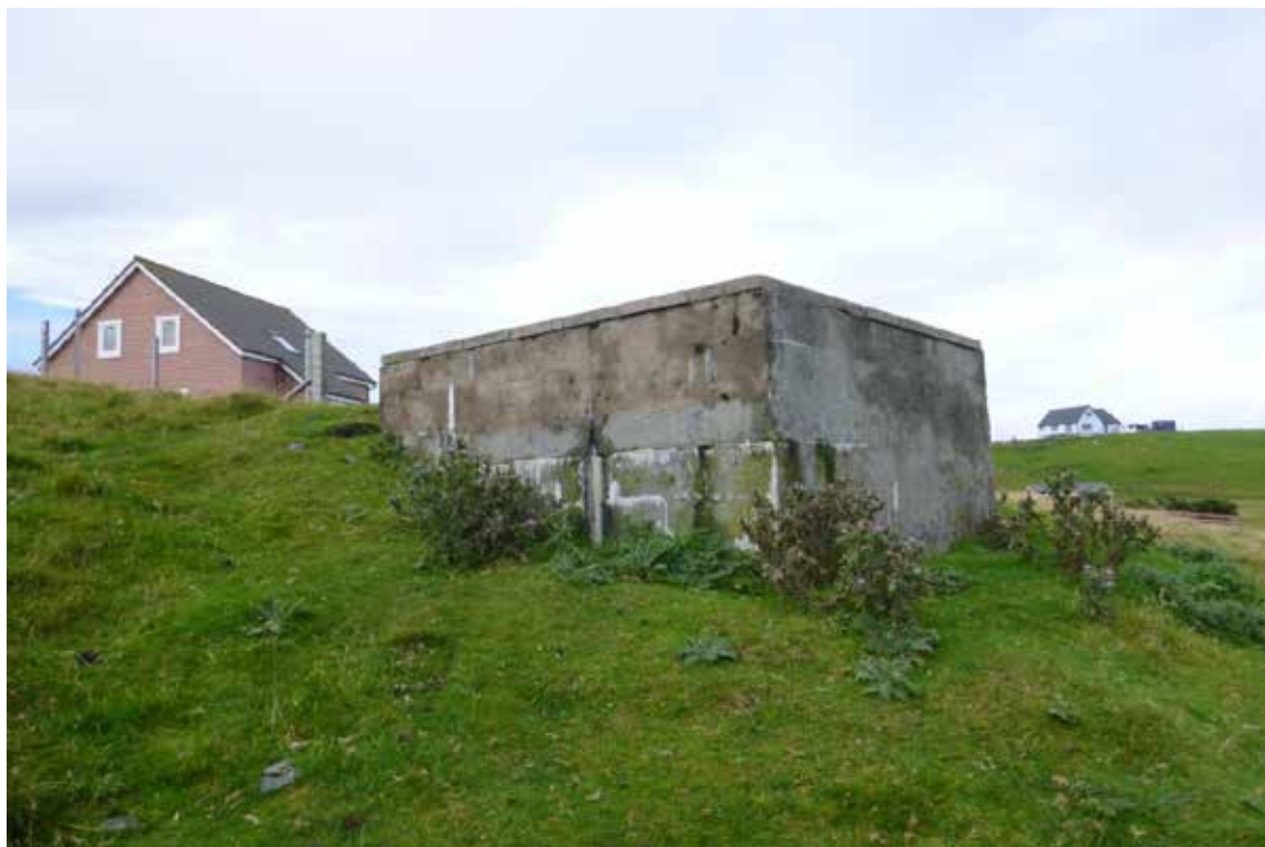
Figure 14 – Septic tank associated with a house in the Glendale area.
