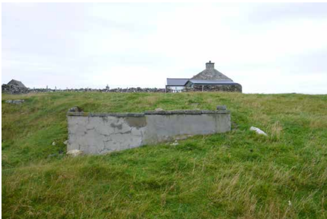
Figure 10 – Concrete septic tank servicing houses in the Wester Quarff area.
