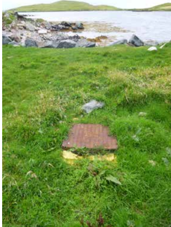
Figure 12 – Man hole cover associated with a septic tank servicing the Scottish Sea Farms Ltd. shore base at the Voe of North House.
