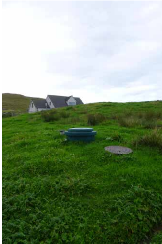
Figure 9 – Plastic septic tank servicing a house in the Wester Quarff area.
