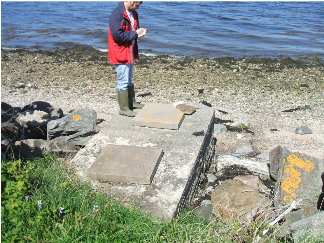
Figure 11. Septic tank at Balblair
