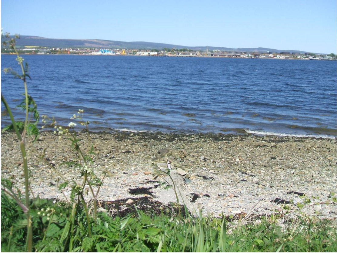
Figure 12. Discharge pipe at Balblair
