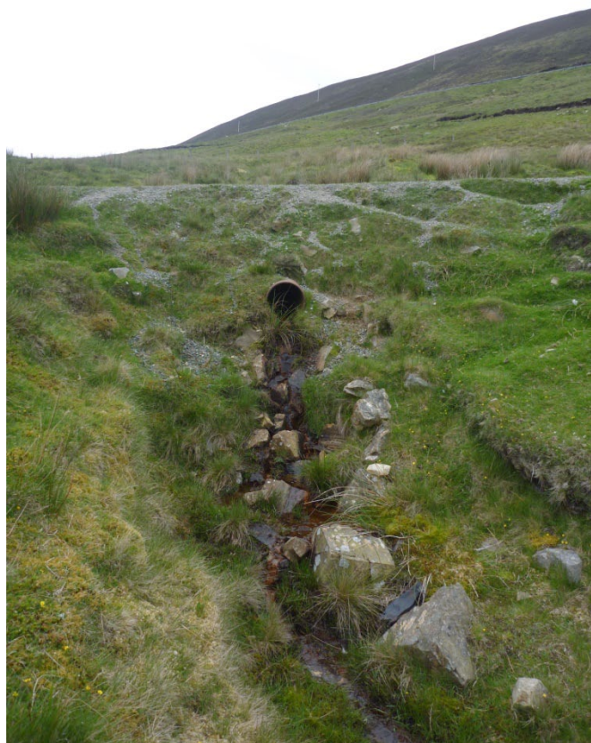
Figure 6. Pipe running under road
