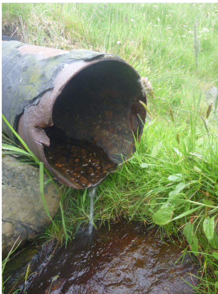
Figure 14. Pipe. Location of fresh water sample Dales Voe FW11
