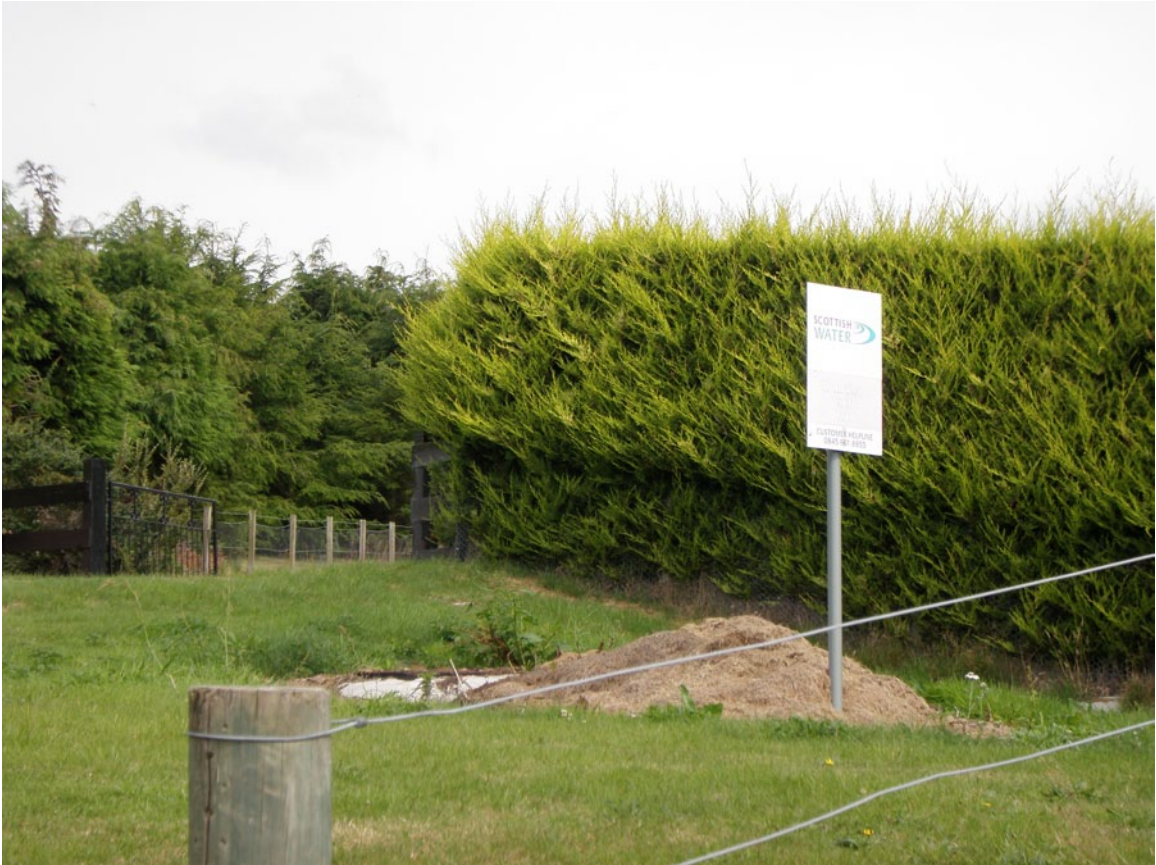
Figure 4. Drumduran septic tank
