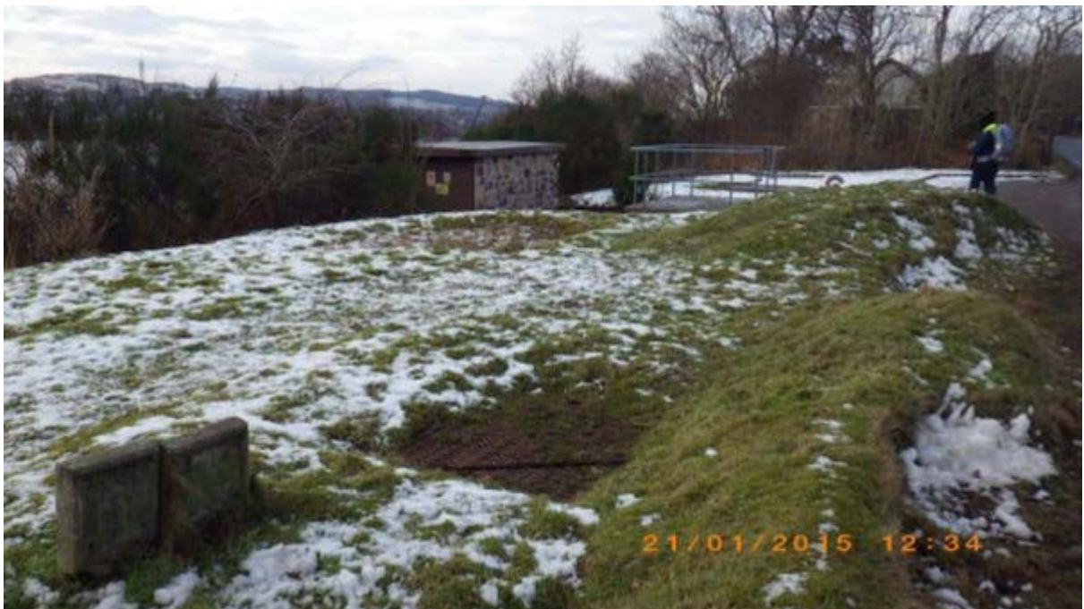
Figure 22. Scottish Water WWPS, North Connel, east of the Connel Bridge. Waypoint 127.
