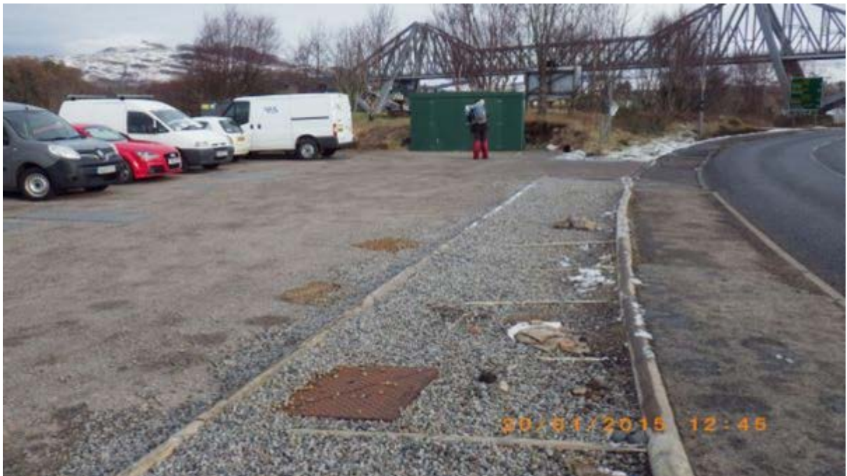
Figure 14. Scottish Water WWPS at south west side of Connel Bridge. Waypoint 68.
