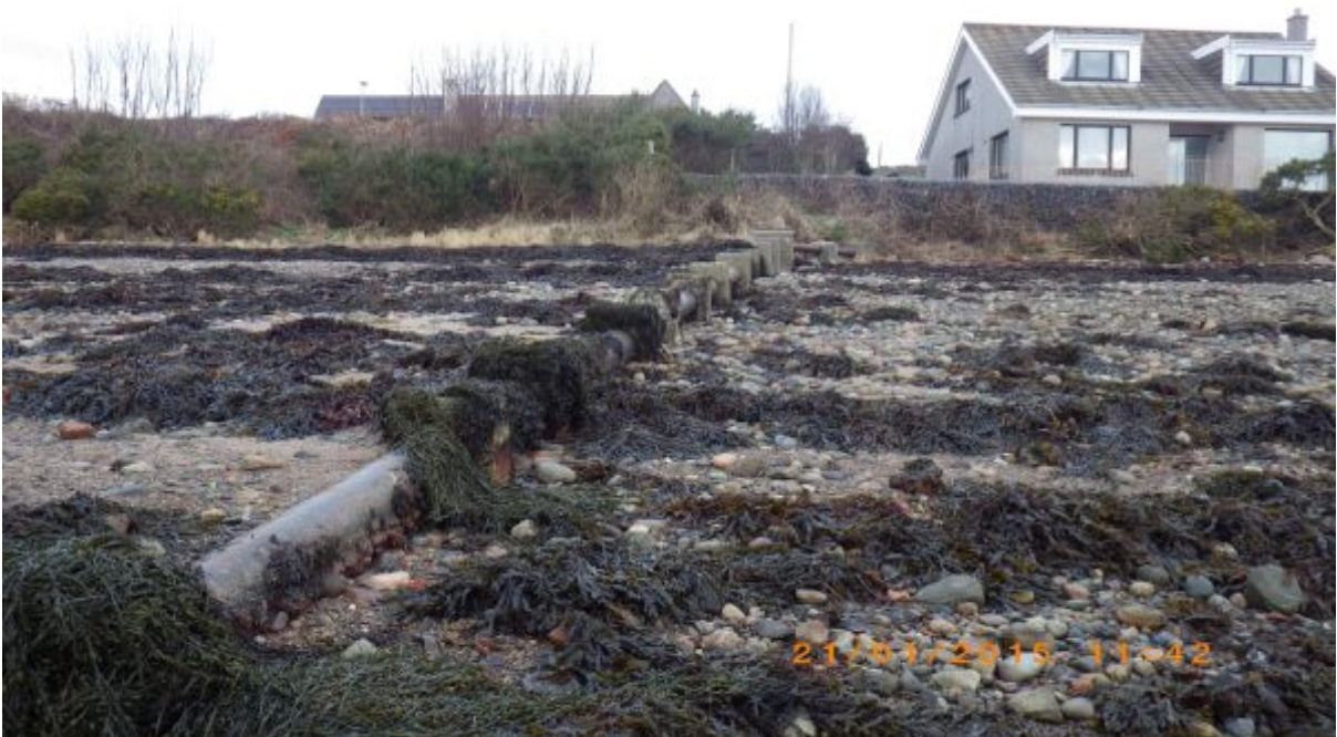
Figure 20. Outfall pipe, North Connel, with end at subtidal level. Watpoint 116.
