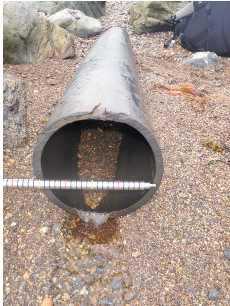
Figure 20 Discharge pipe at Aith
