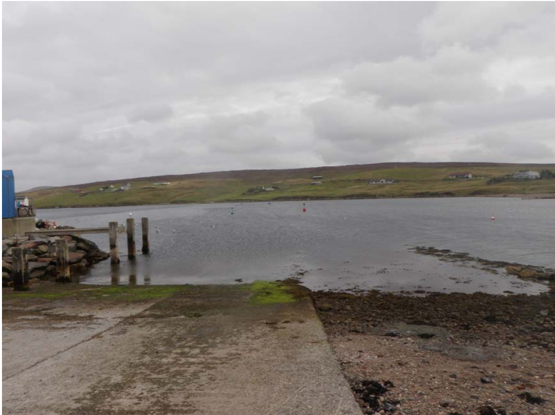
Figure 8. Slipway adjacent to the lifeboat station at Aith.
