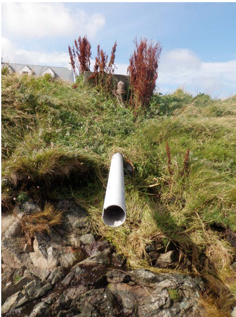
Figure 15. Dry pipe from septic tank.
