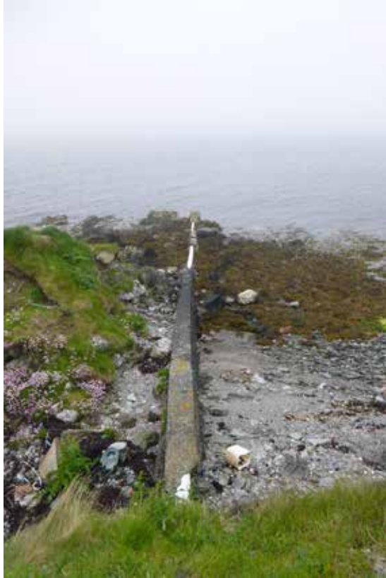
Figure 14 – Discharge pipe from septic tank in Figure 13. Seawater sample obtained from shore.
