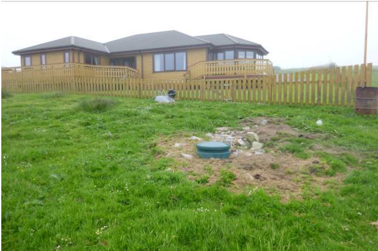
Figure 10 – A second septic tank associated with houses at Scarfataing
