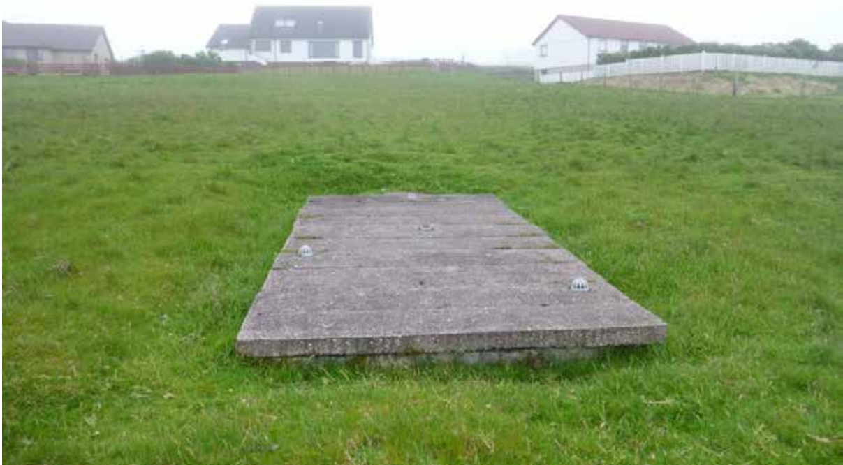
Figure 12 – Concrete septic tank below a group of houses near Cauldhame.
