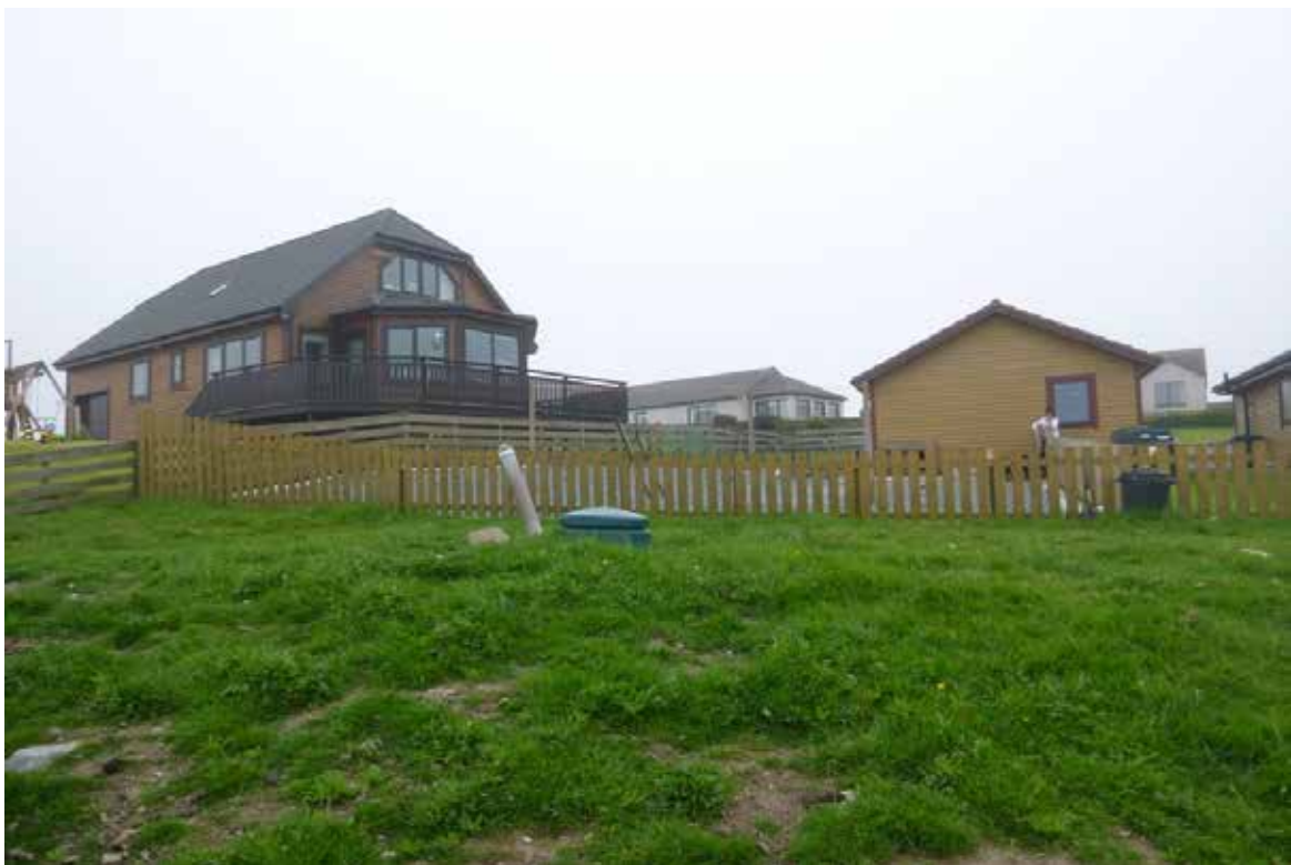
Figure 9 – Septic tank associated with houses at Scarfataing
