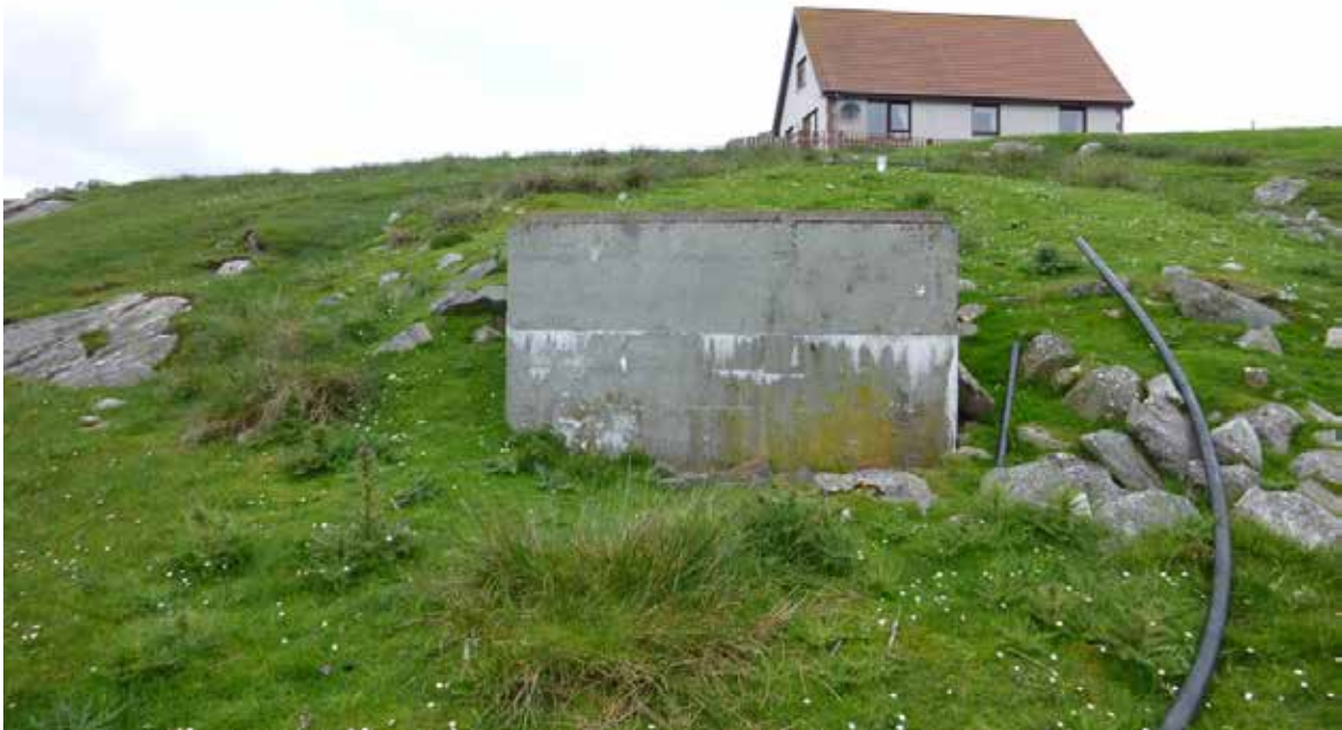
Figure 6 – Septic tank associated with a house at Burwick
