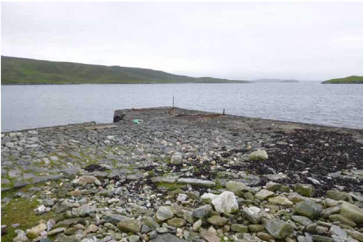
Figure 17 – Small stone pier at the Ness of Burwick
