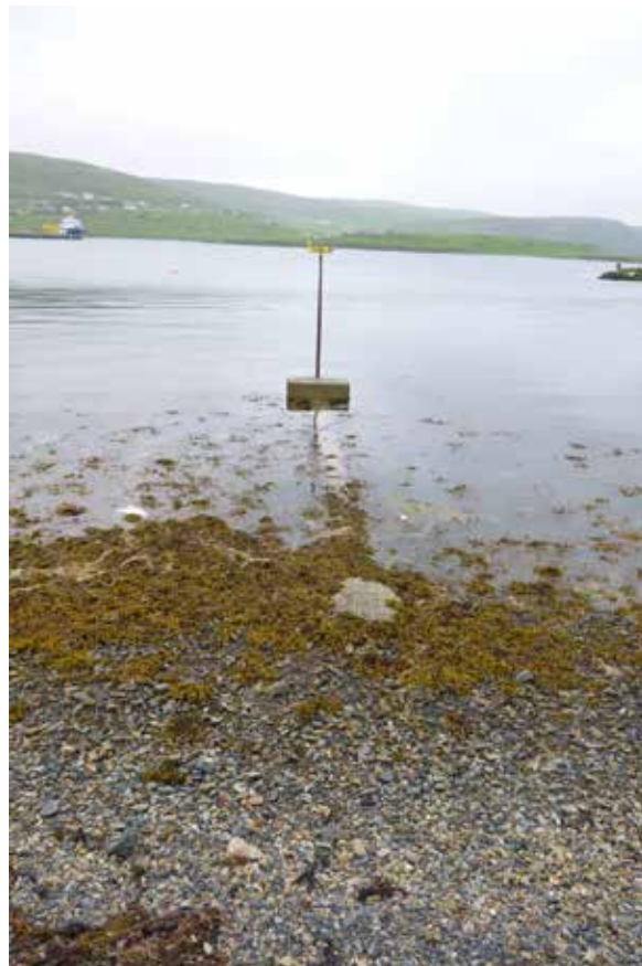
Figure 7 – Pipe associated with the West Shore Sewage Pumping Station
