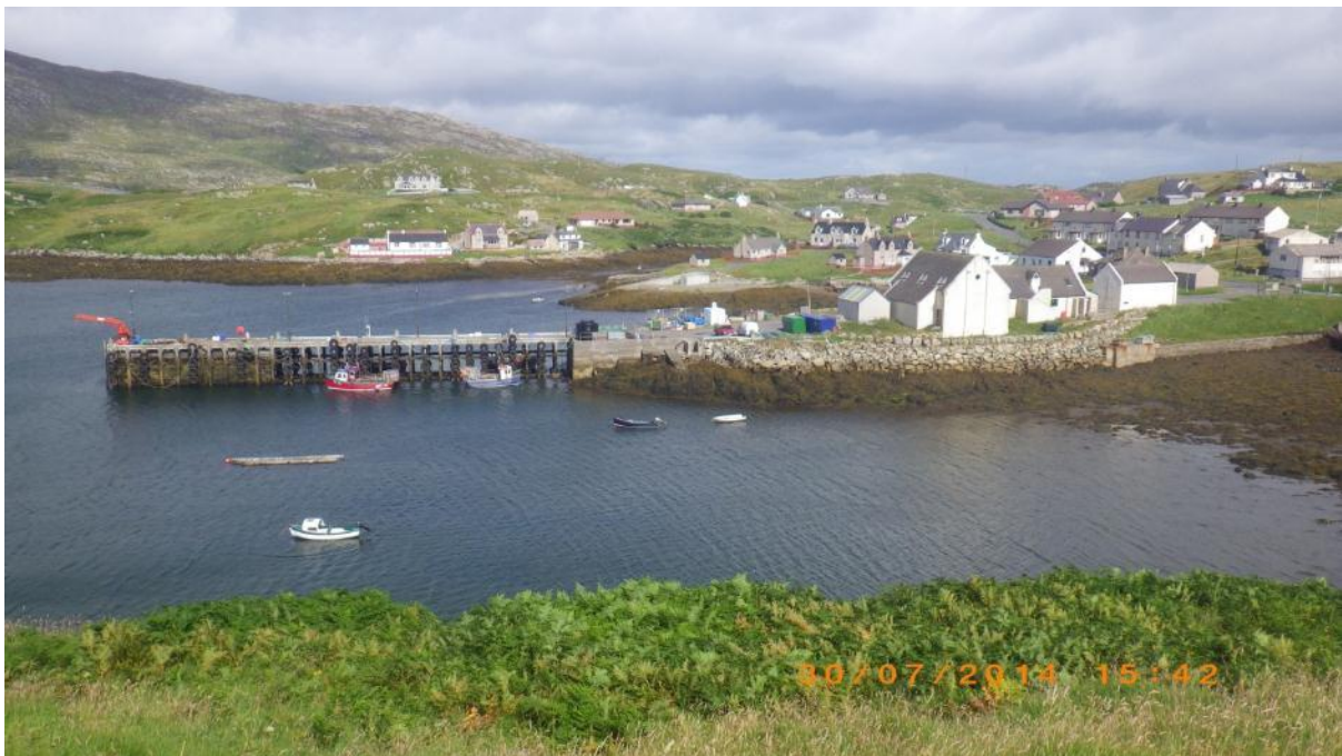
Figure 12. Overview of Scalpay harbour area looking north with the two harbours, either side of the pier. Cenn a' Bhaigh middle distance, partially hidden. Waypoint 45.
