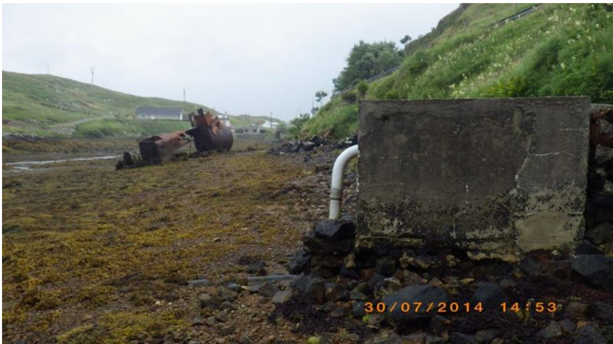
Fig. 10. Disused septic tank with broken outfall pipe south side of Ceann a Bhaigh. Large rusting marine metal fragments onshore in the background looking east. Waypoint 35.
