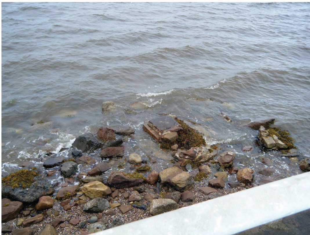
Figure 10. Manhole cover on shore
