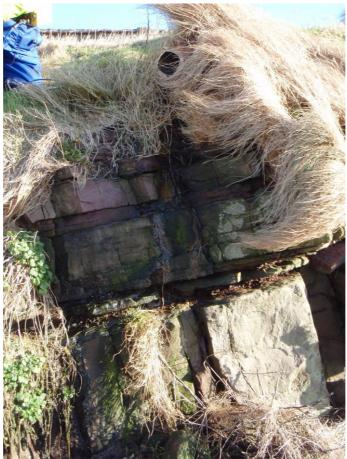
Figure 4 15cm pipe flowing from cliff onto shoreline. Mulched toilet tissue in pile underneath pipe.
