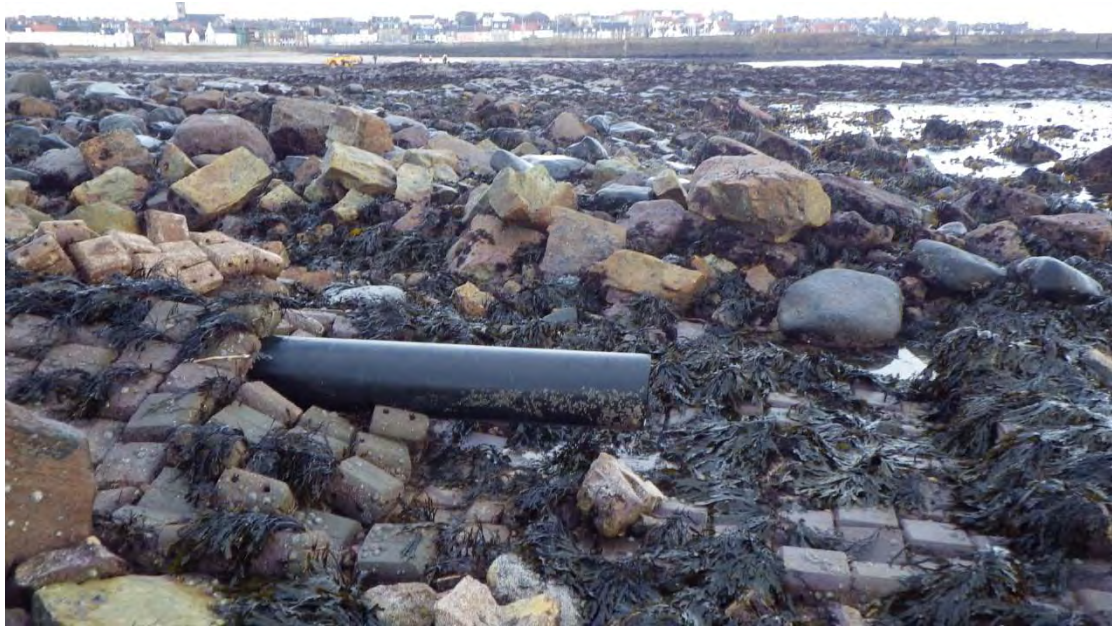
Figure 6. End of outfall pipe (Waypoint 3, ANS2)
