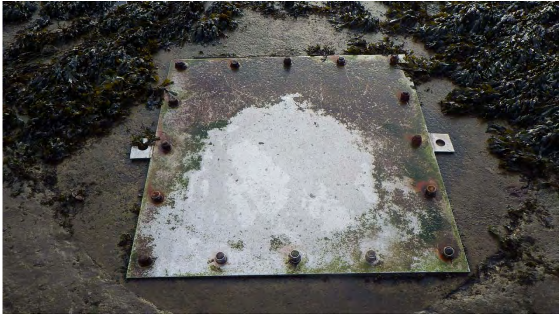
Figure 14. Manhole cover on shoreline (Waypoint 10)
