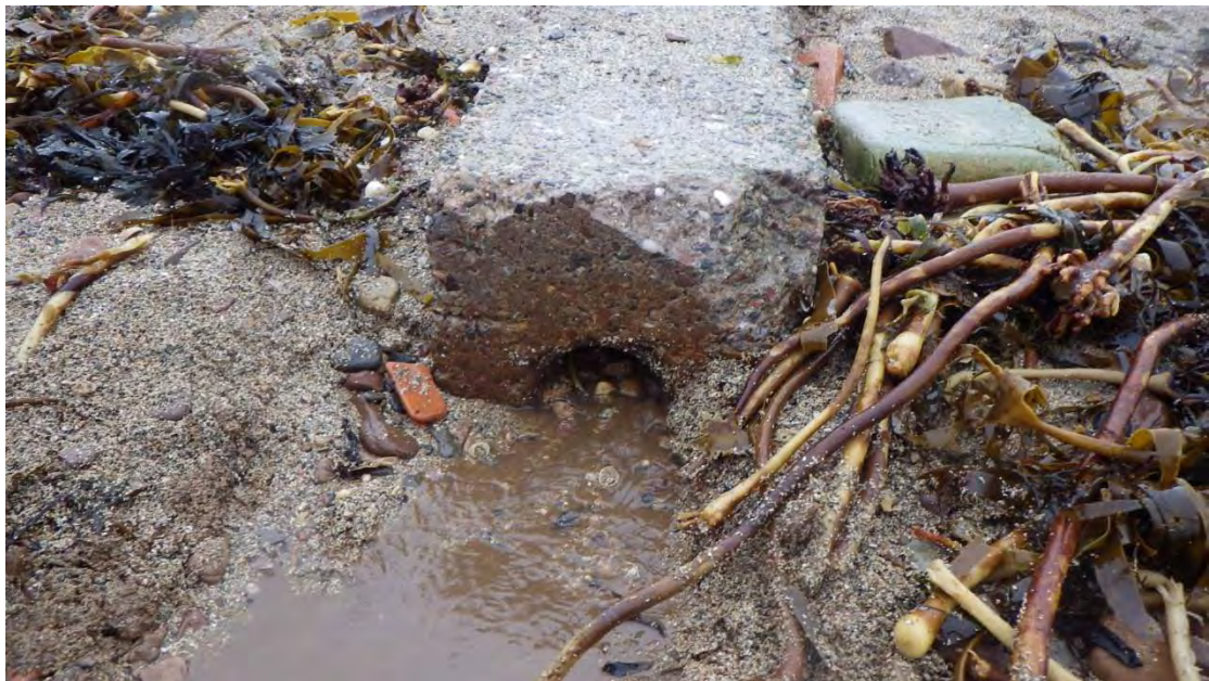
Figure 21. Old concrete pipe, possibly land drain from pig farm (Waypoint 16)
