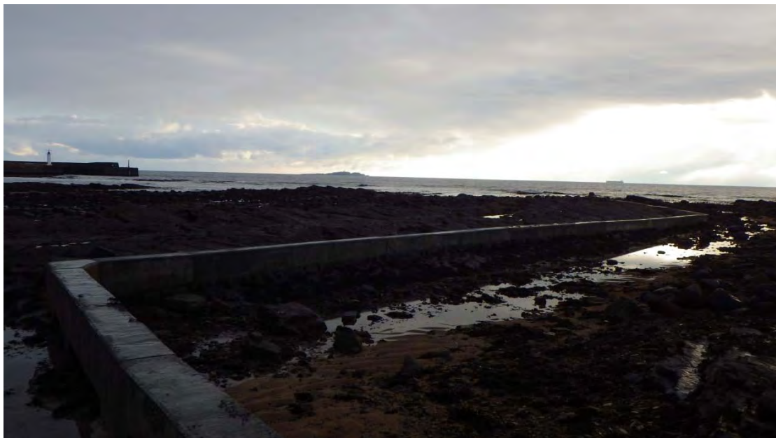
Figure 5. Sewage outfall pipe in Anstruther bay (WP2)
