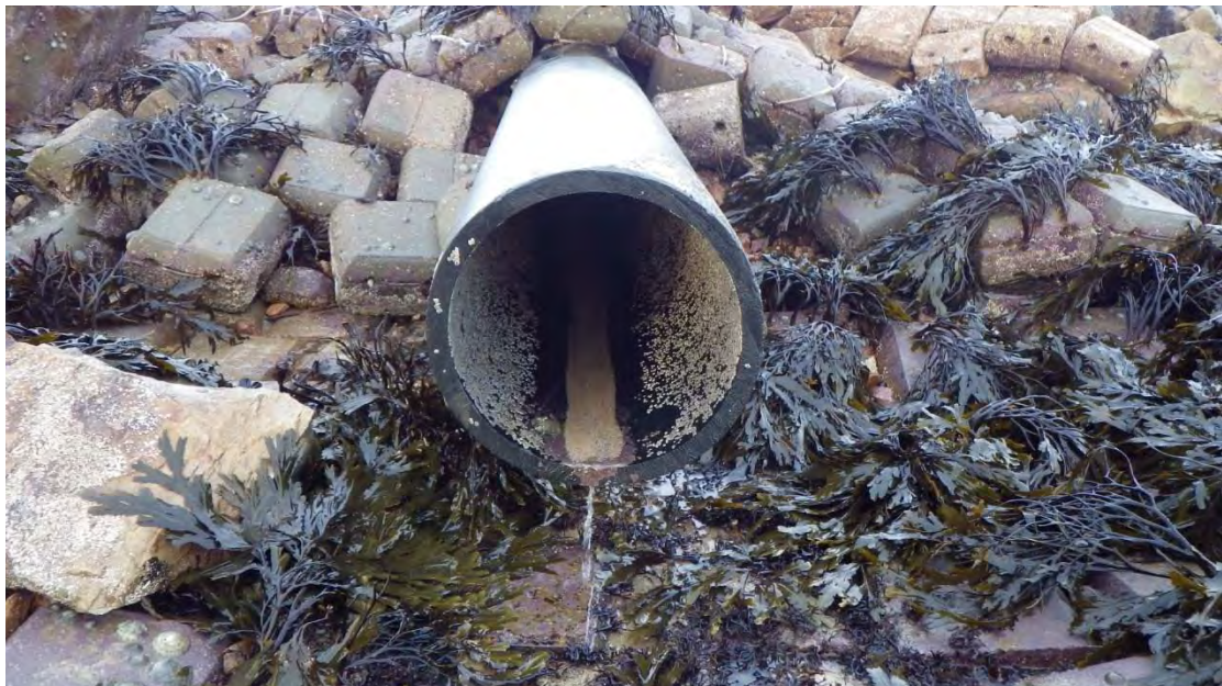
Figure 7. End of outfall pipe (Waypoint 3, ANS2)
