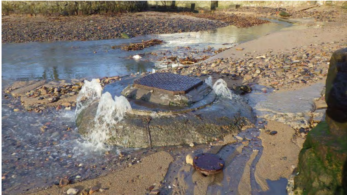
Figure 10. Dreel Burn with overflowing sewage drain next to it (Waypoint 5, ANS3)
