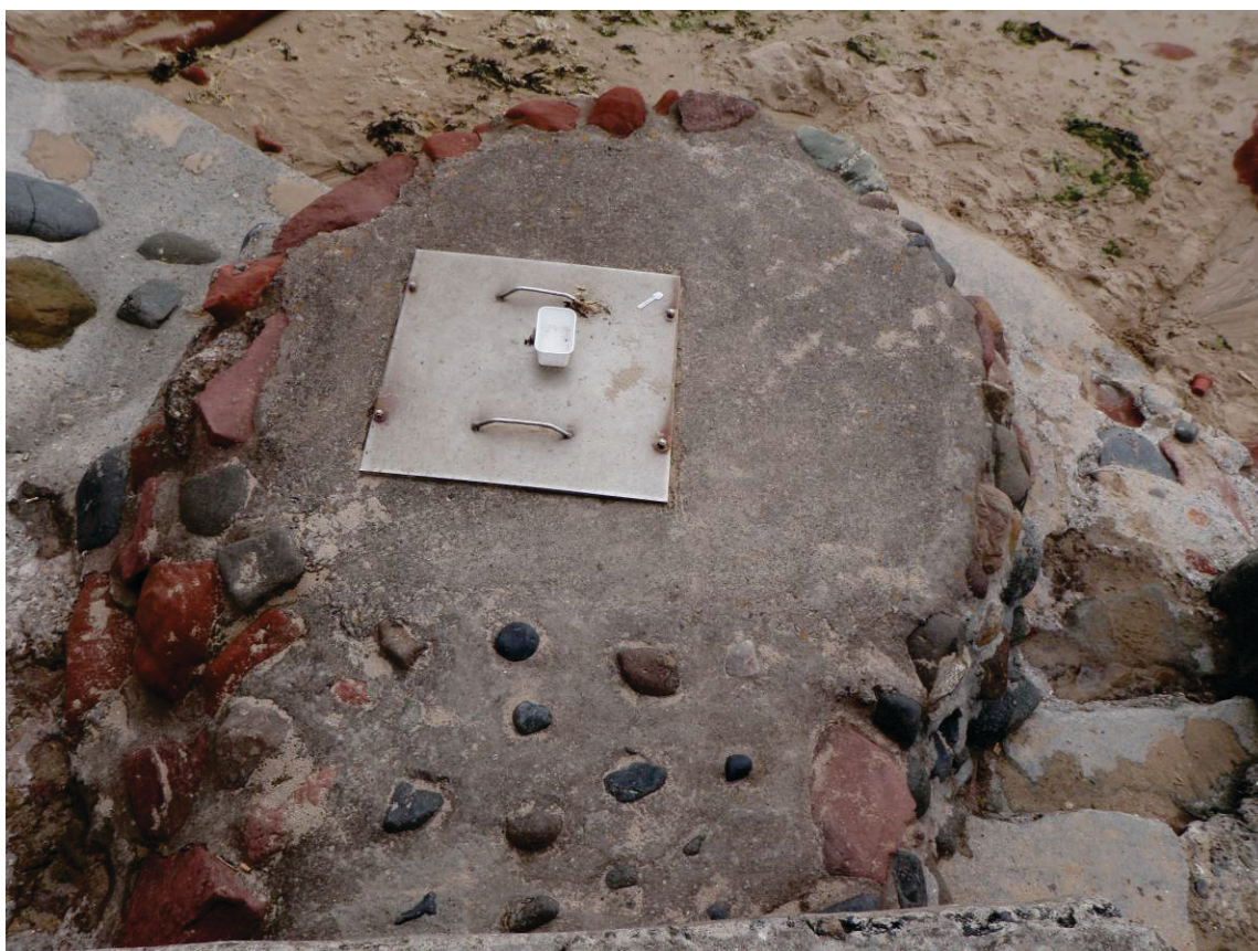
Figure 18. Inspection cover, no sign of outfall pipe
