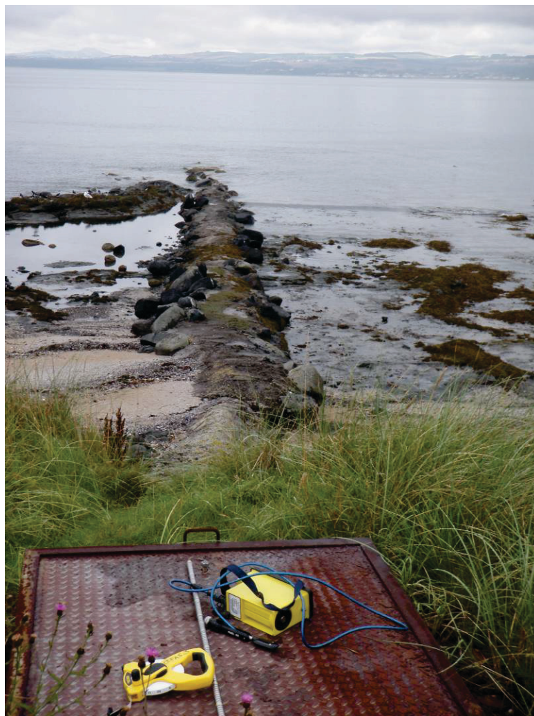
Figure 10. Inspection cover & outfall pipe. Also location of sea water sample (LBSW5)
