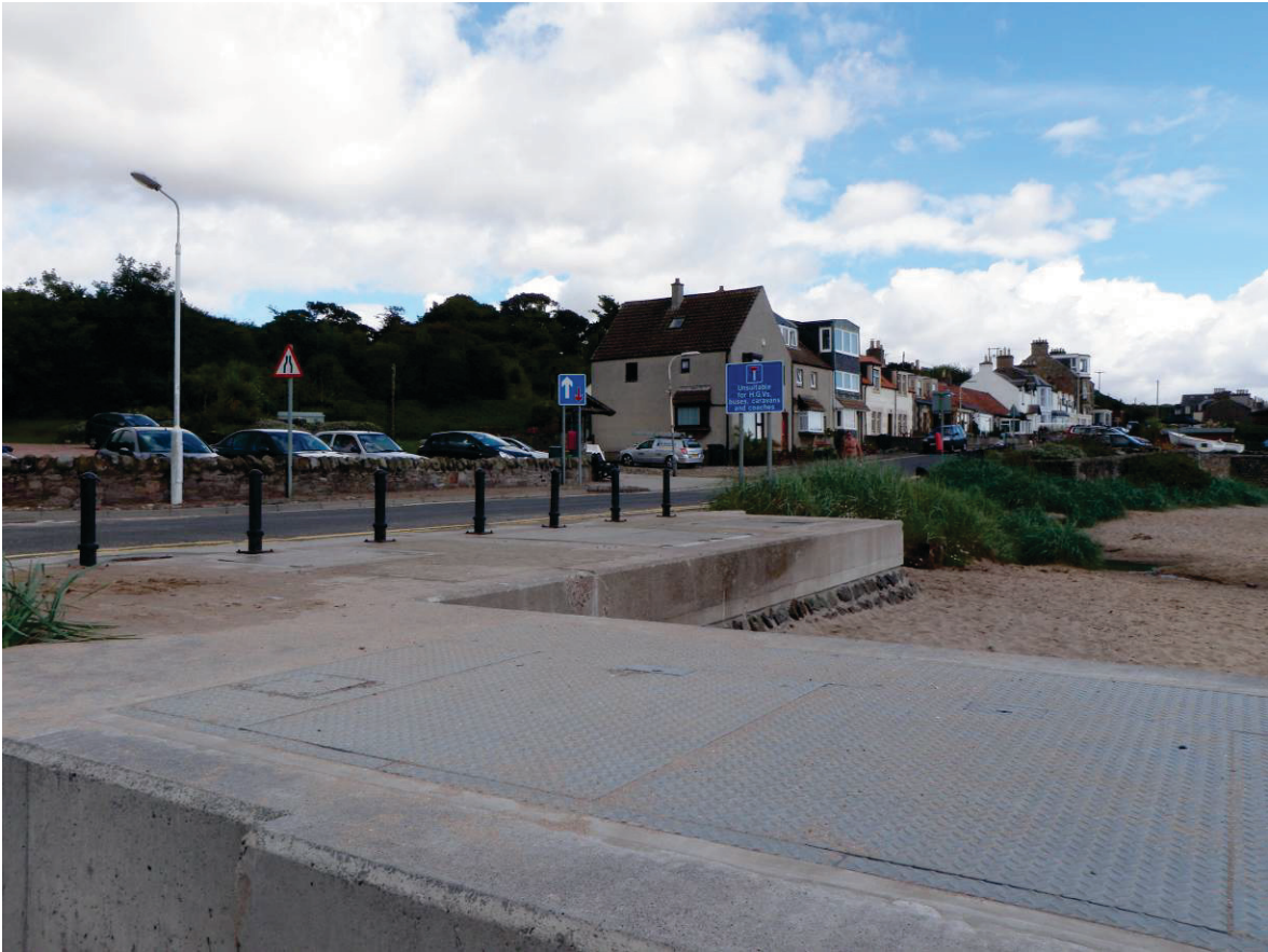
Figure 16. Septic tanks/pumping station
