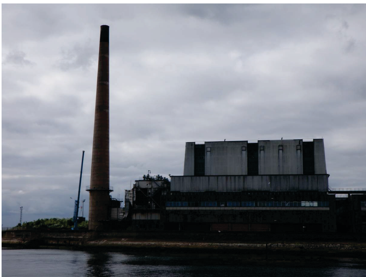
Figure 29. Abandoned power station
