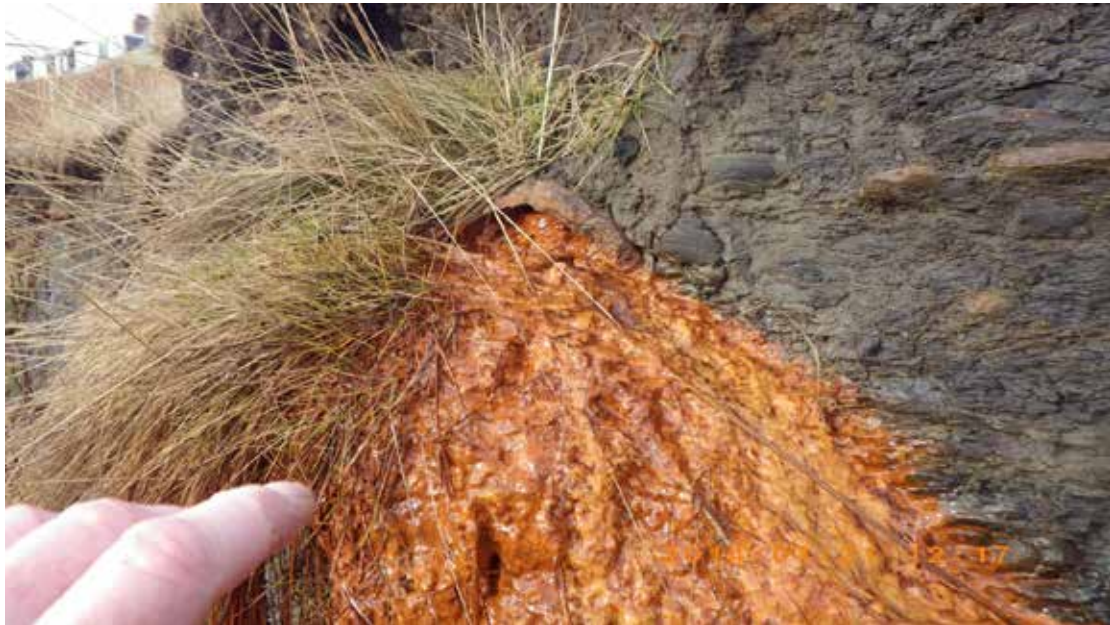
Figure 13. Old iron pipe, partially blocked with stained deposit below. Associated with waypoint 25 and sample FWFEP3
