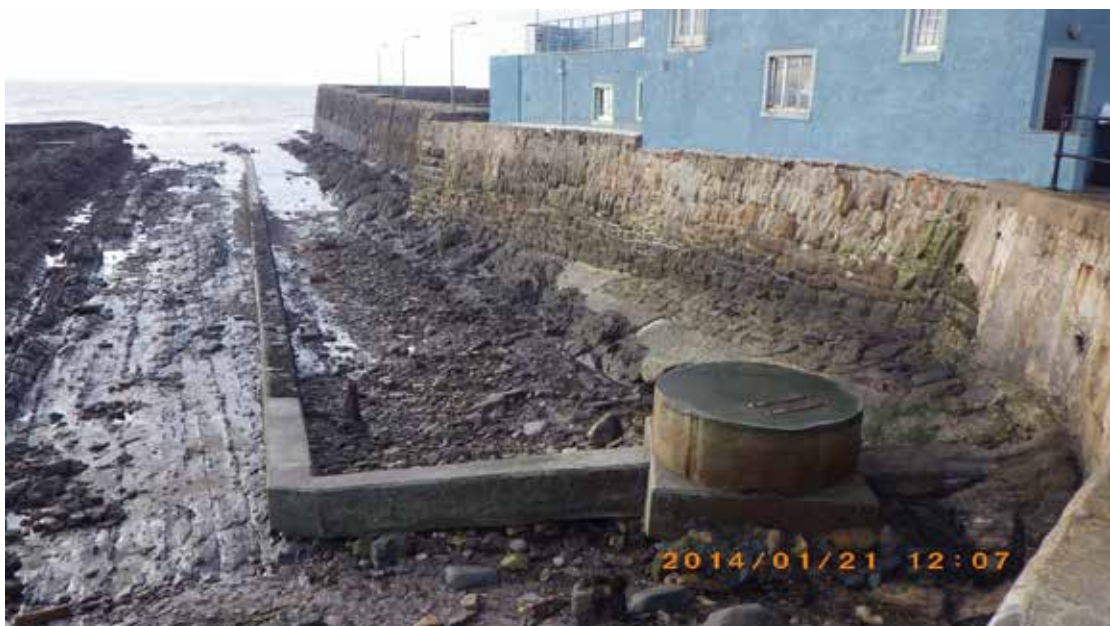
Figure 12. Large pipe in concrete casing on lower shore issuing from circular concrete inspection unit with manhole access cover. Associated with waypoint 23
