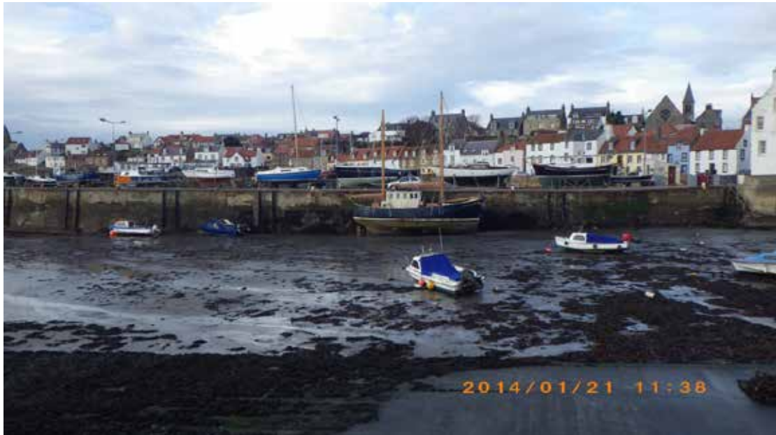
Figure 11. East harbour at St Monans. Associated with waypoint 20
