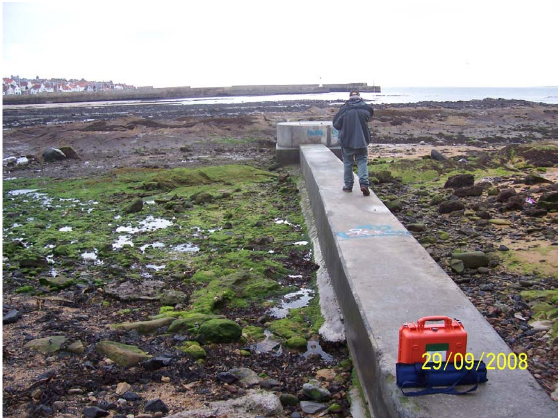
Figure 15. Unknown outlet (new construction, no flow)
