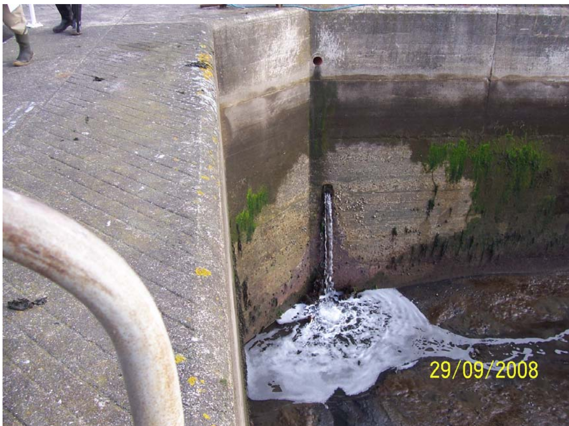
Figure 8. Outfall pipe (Inaccessible)
