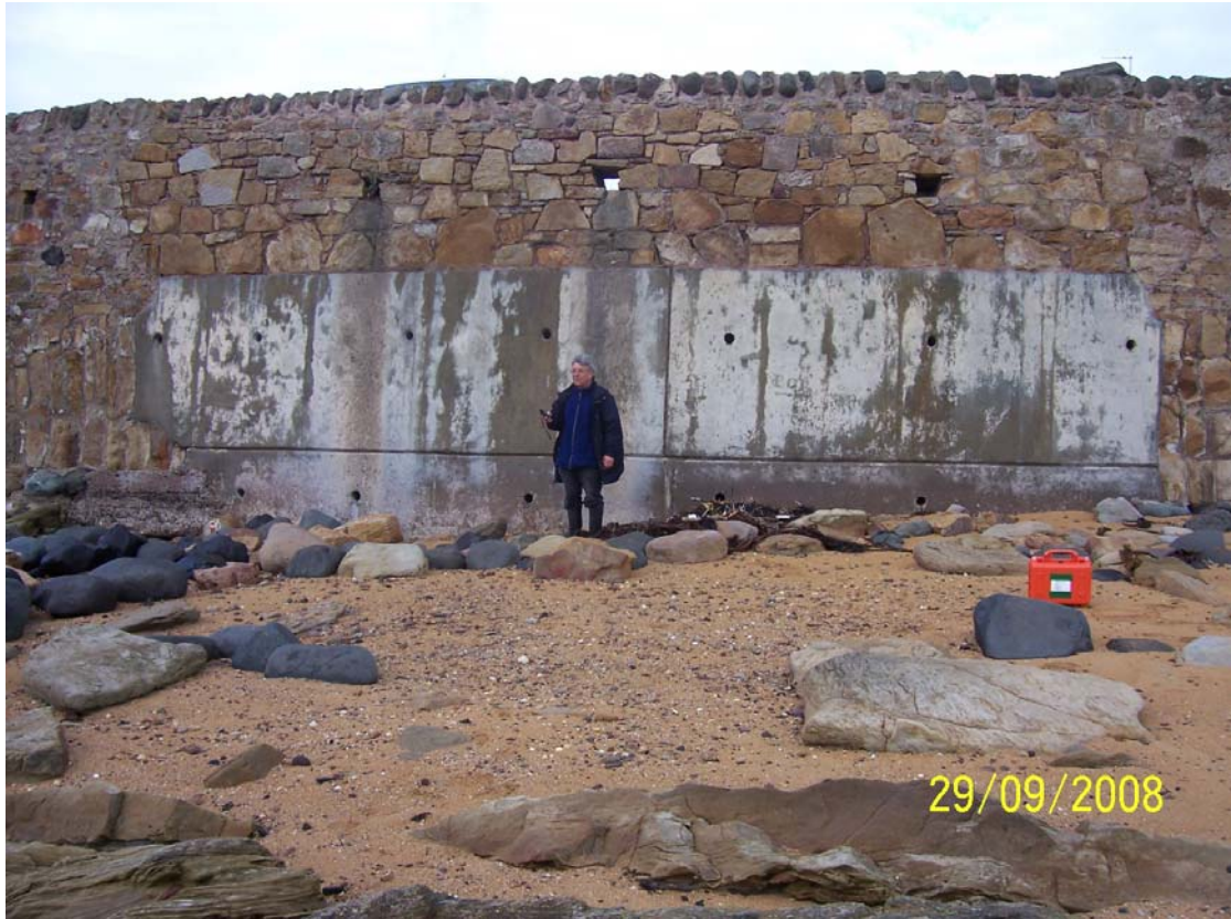
Figure 17. Drainage holes in wall below golf course car park
