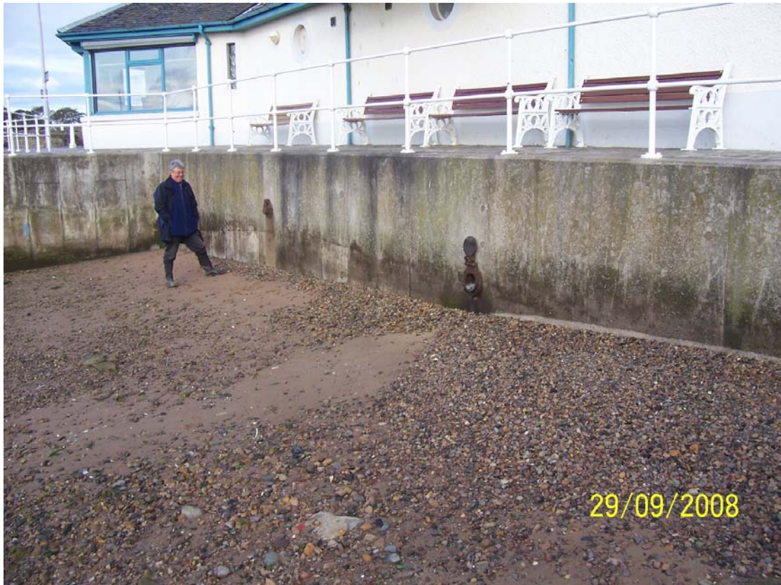
Figure 9. Outfall pipe below public toilets
