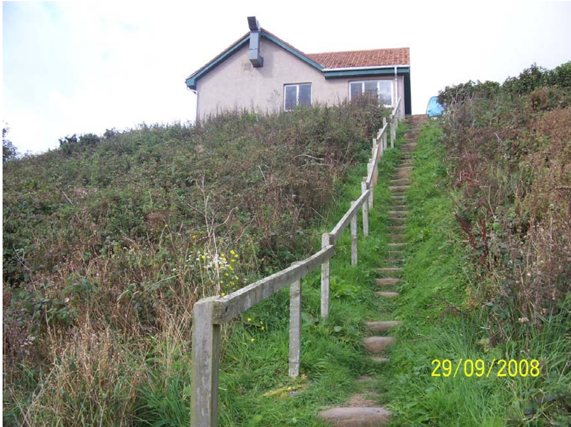
Figure 34. St Monans pumping station
