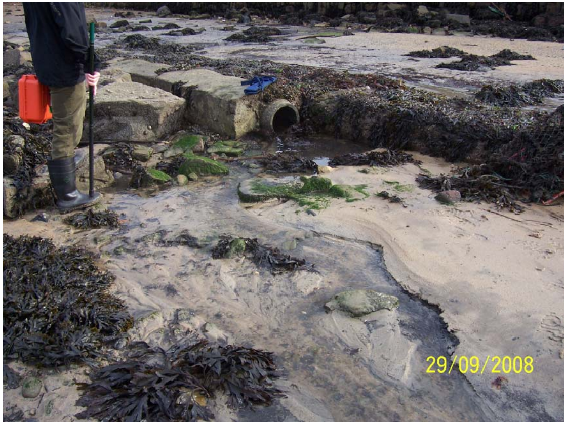
Figure 11. Outfall pipe on shoreline (Water sample 2)
