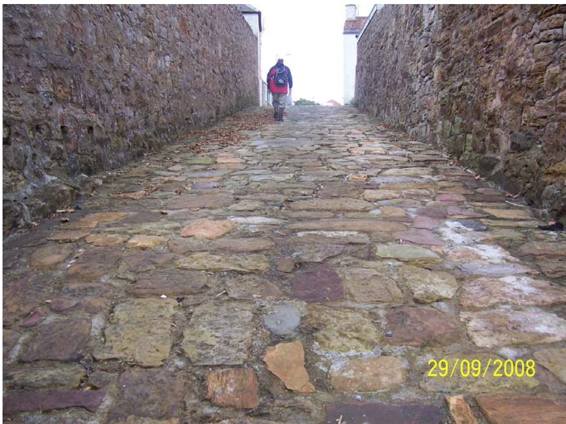
Figure 14. Slipway and evidence of runoff
