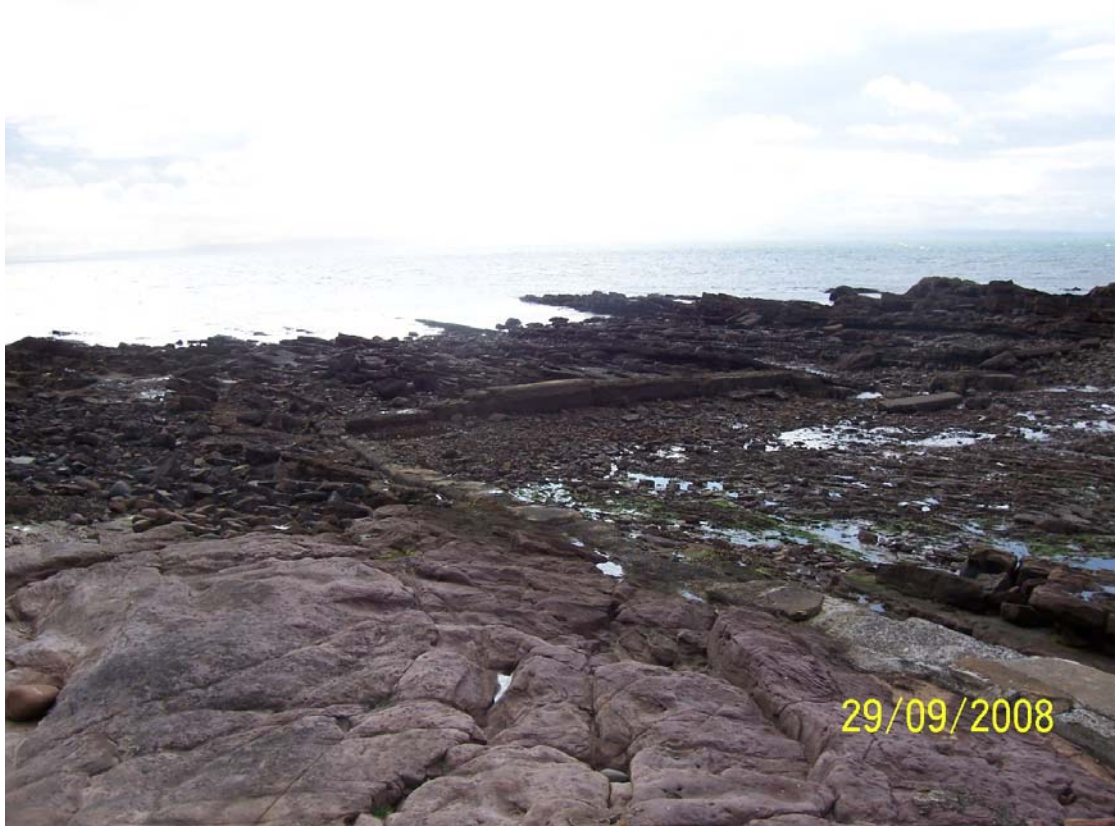
Figure 20. Old and inaccessible outfall pipe
