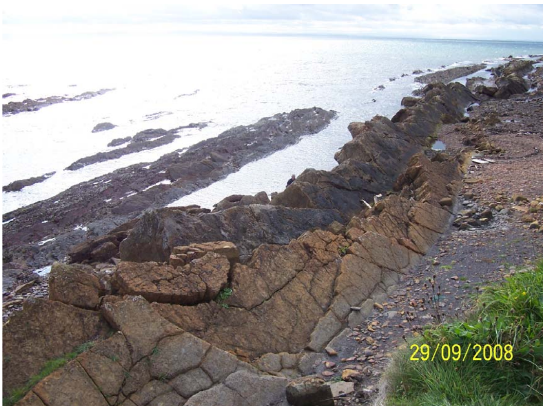
Figure 35. Location of seawater sample 7 near St Monans pumping station
