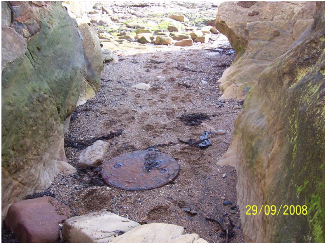
Figure 27. Manhole cover associated with outfall pipe in Figure 38
