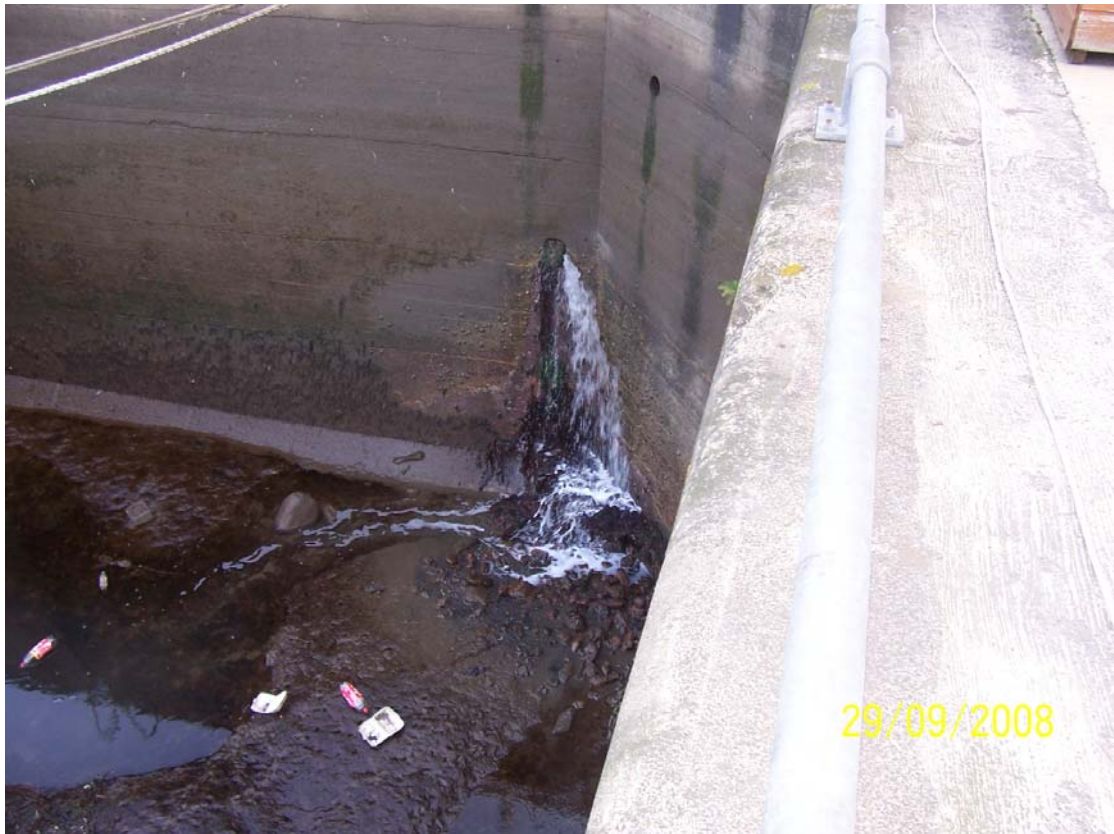
Figure 7. Outfall pipe (Inaccessible)
