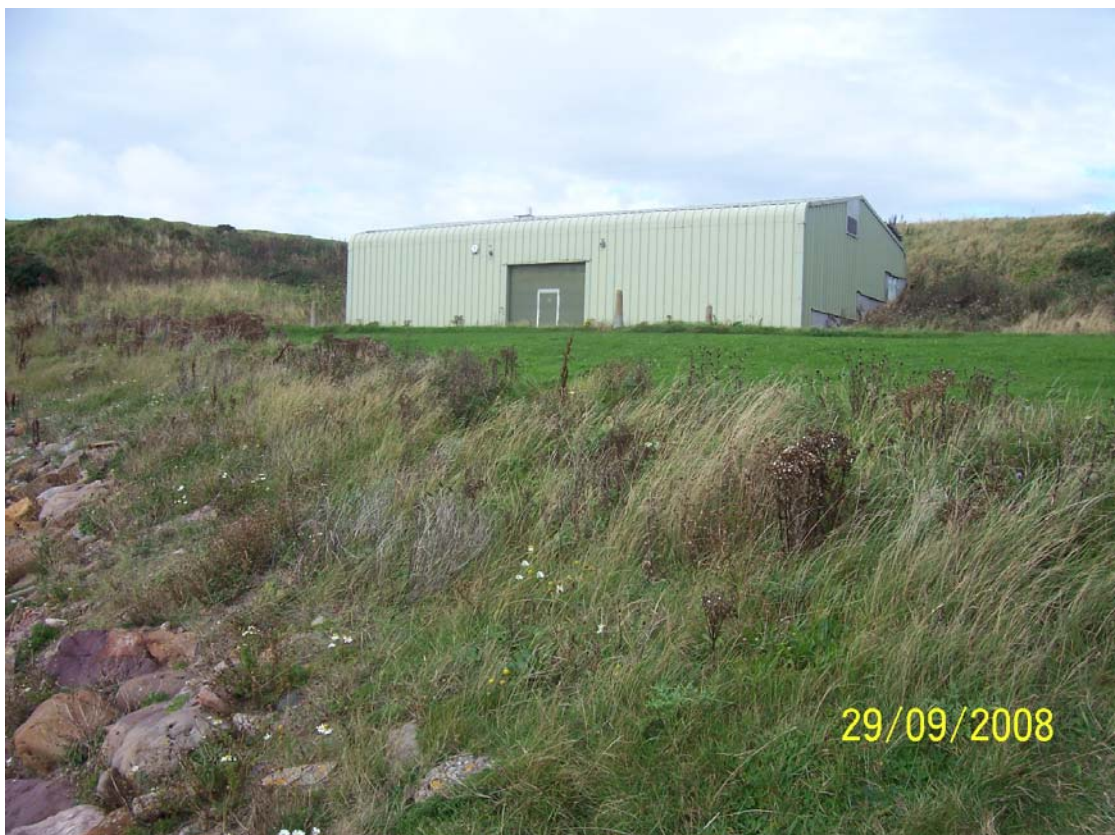
Figure 18. Sewage pumping station
