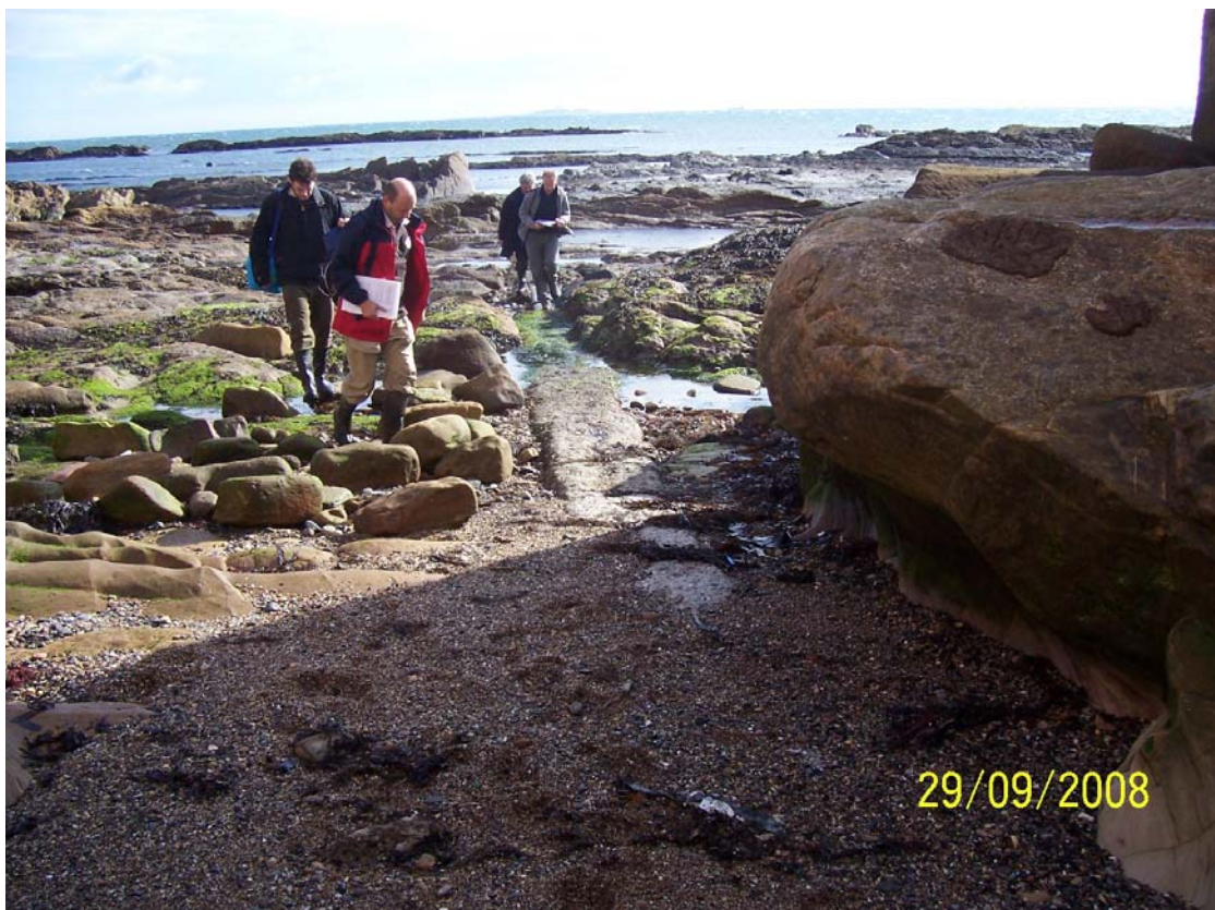
Figure 26. Unknown pipeline, no obvious outfall due to incoming tide
