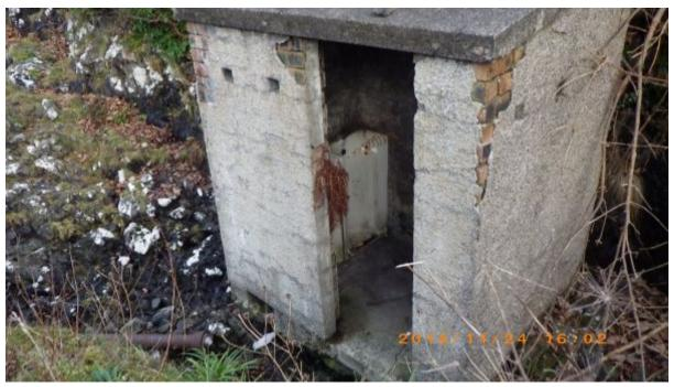
Figure 14. Disused urinal with metal outflow pipe associated with wp 34.
