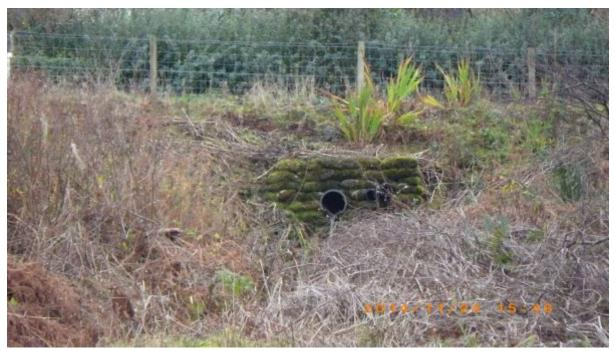
Figure 13. Watercourse diverted under road via pipe associated with wp 33.
