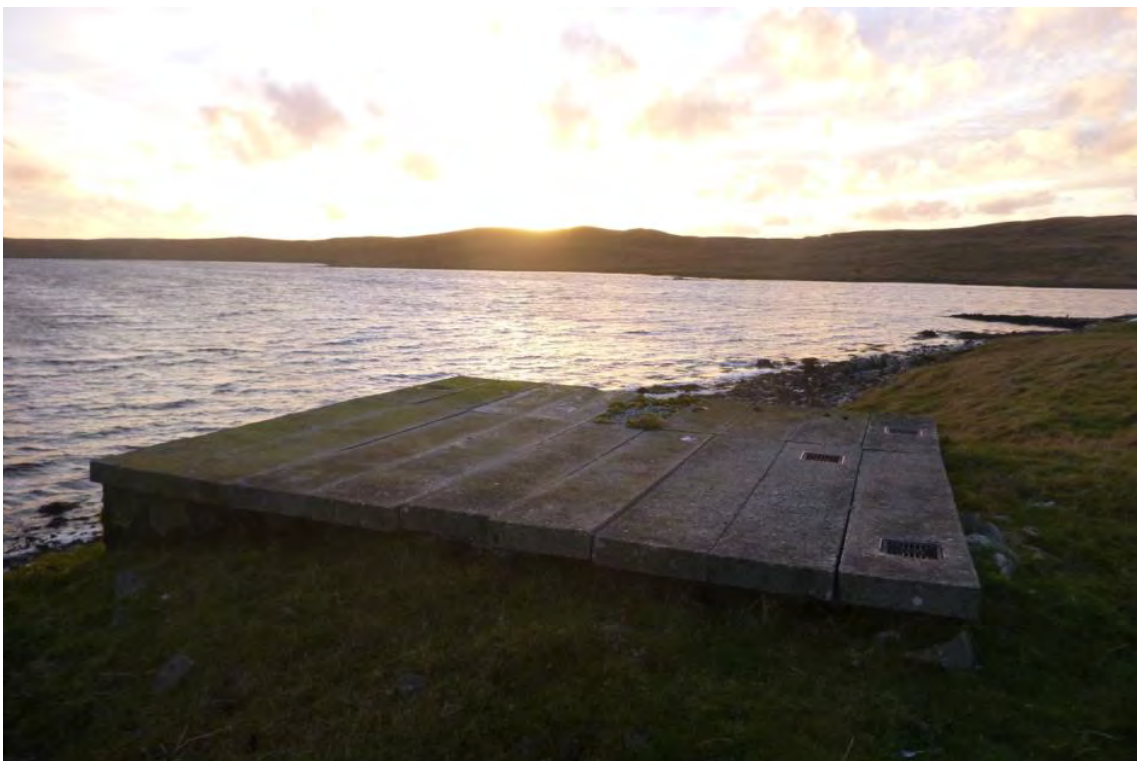
Figure 15 – Concrete septic tank near shoreline below chalet at Bridge of Walls.
