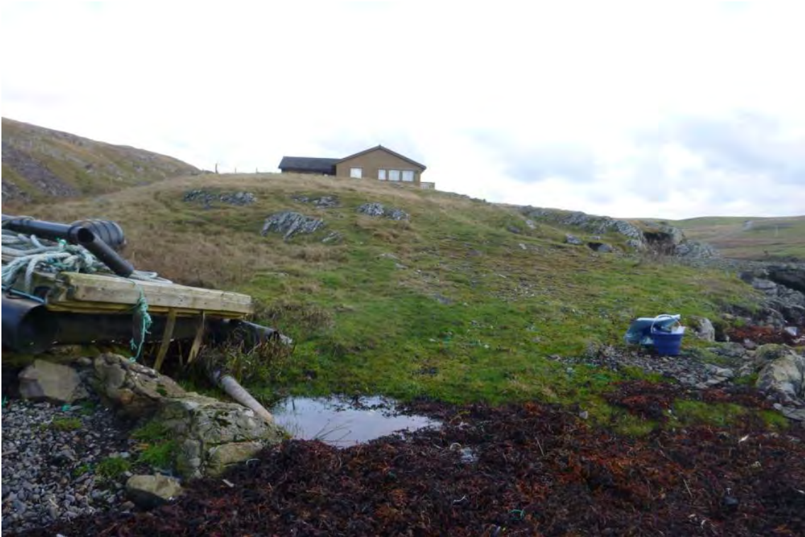
Figure 10 – Position of pipe (in figure 9) in relation to dwelling house.
