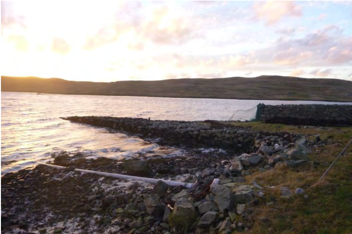
Figure 16 – Outlet pipe to sea below dwelling house at Bridge of Walls.
