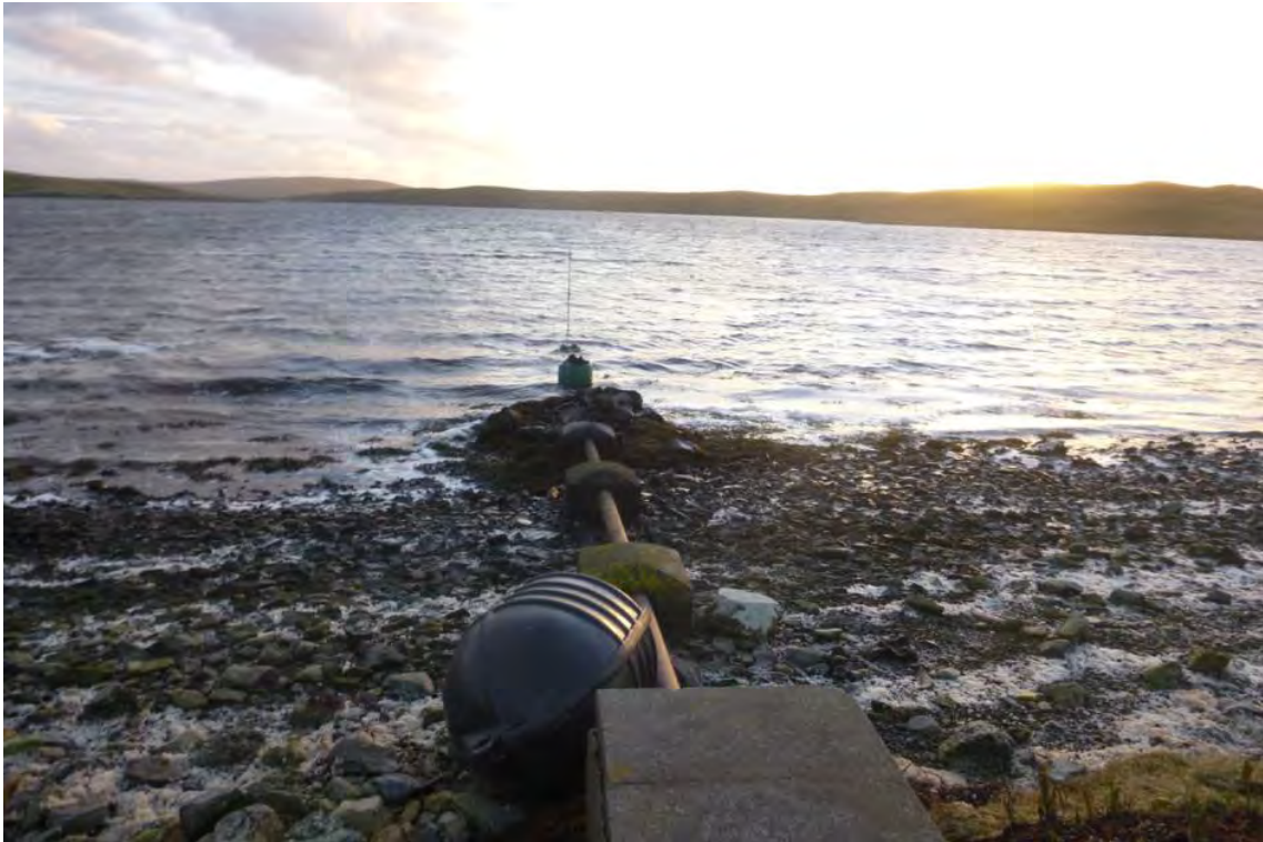
Figure 14 – Outlet pipe to sea below one house at Bridge of Walls.
