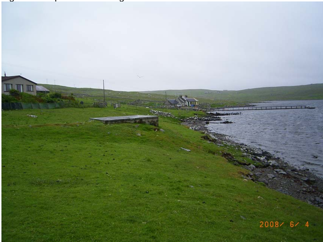
Figure 6. Septic tank at Bridge of Walls
