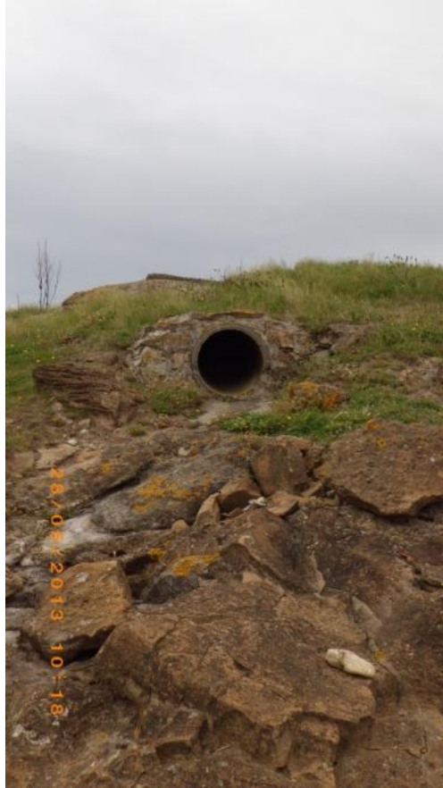
Figure 6. Concrete pipe on shore with metal drain cover sitting above. No flow at time of survey but running water audible. Associated with waypoint 1.
