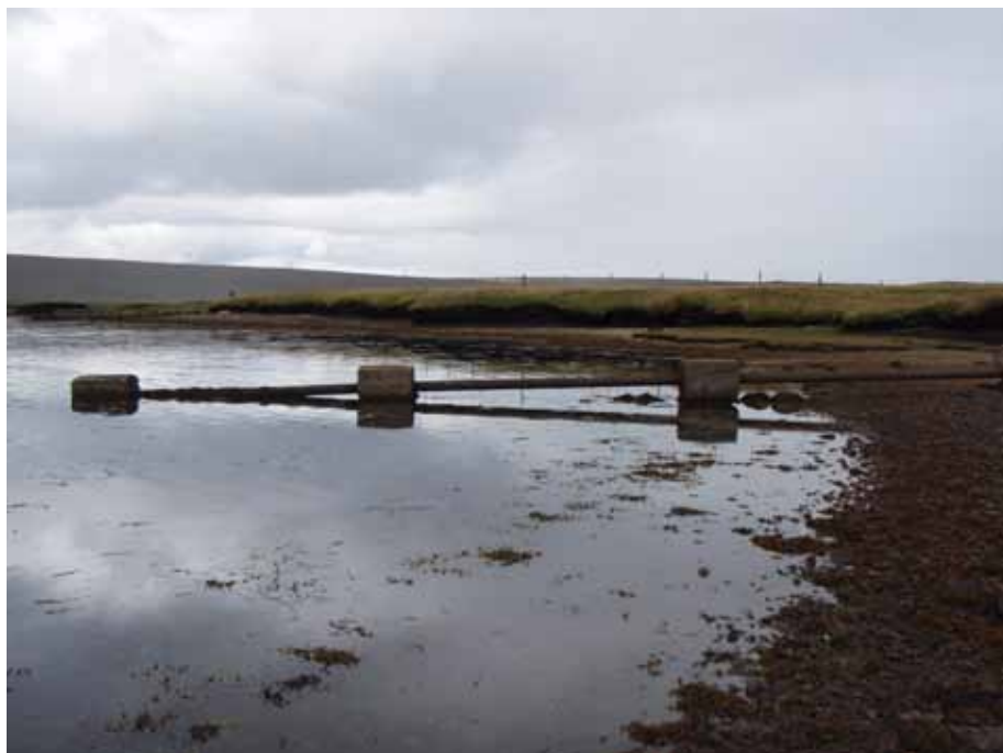
Figure 10. Outfall pipe leading down from houses, location of seawater sample HVSW5
