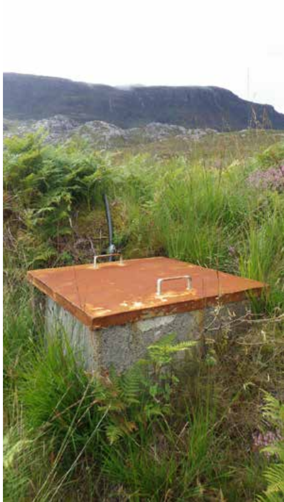
Figure 17: Concrete box with pipe entering, noted on west bank of River Balgy. Waypoint 65
