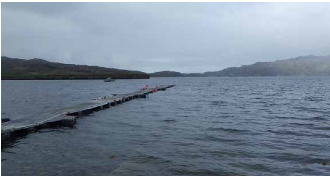
Figure 18: Inner Loch Torridon Marine Harvest shore base, with pontoon and moorings visible. Waypoint 67.
