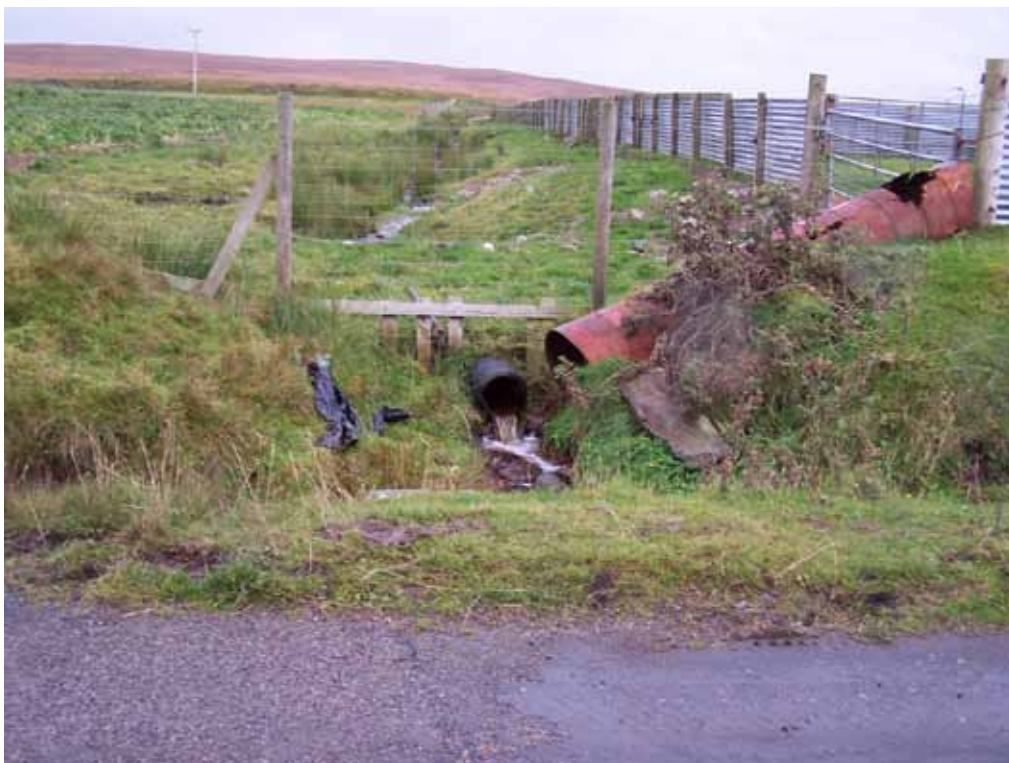
Figure 7 Stream running through metal pipe.
