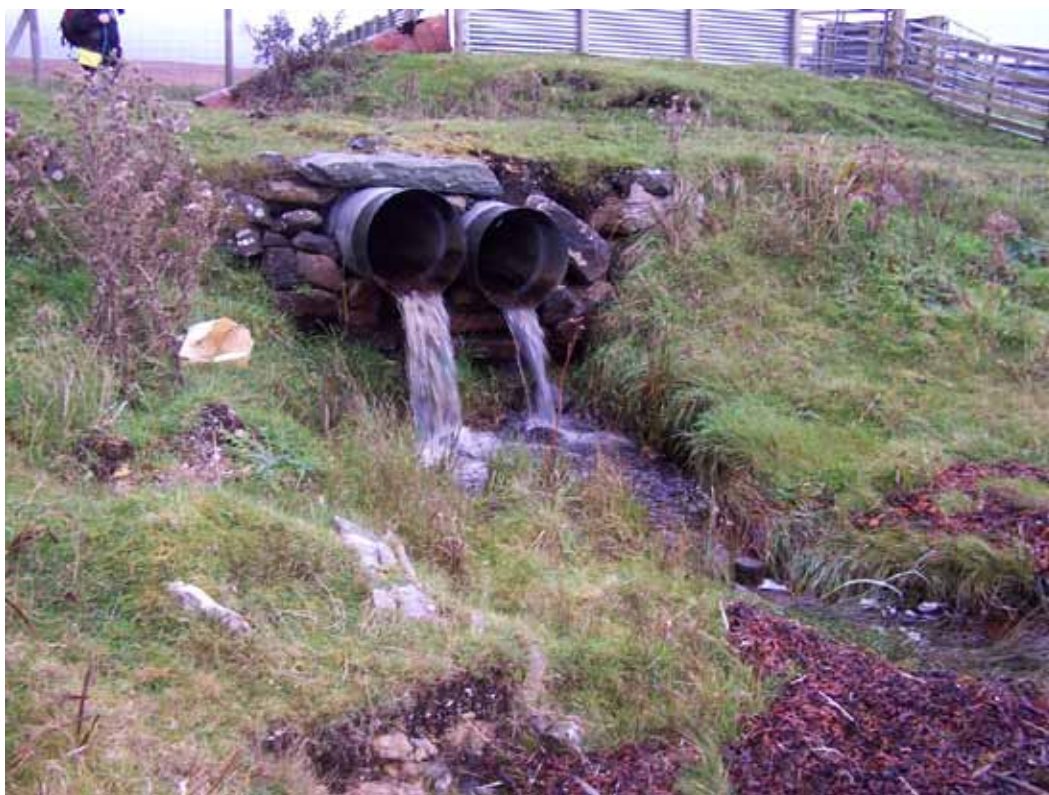
Figure 8 Same stream as above channelled into two metal pipes. Water sample ISW9.
